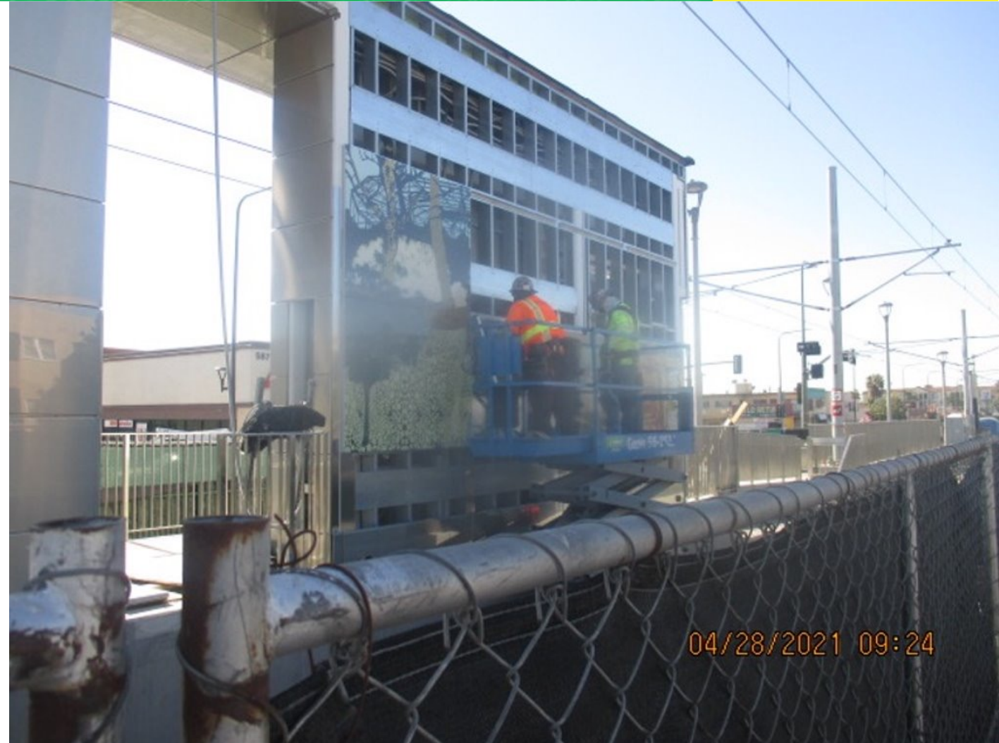
Artwork panel installation at Hyde Park Station
