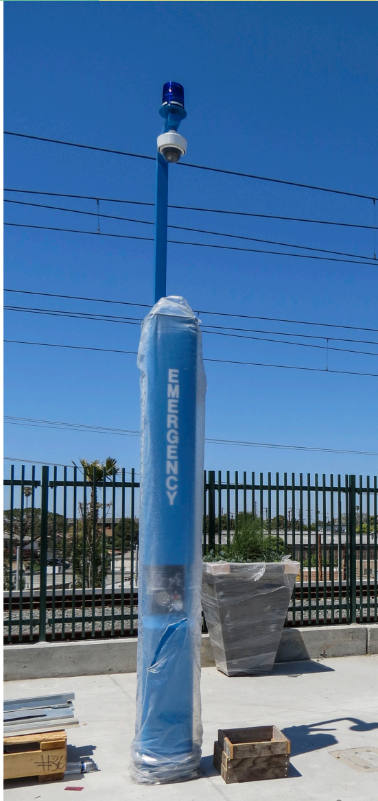
Newly installed CCTV and ETEL with blue light station
