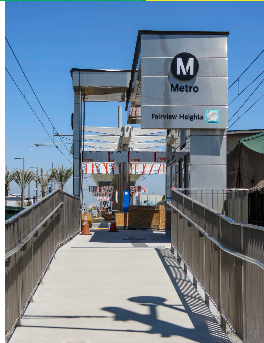
Pedestrian crosswalk, steel bollards, TVM canopy structure
