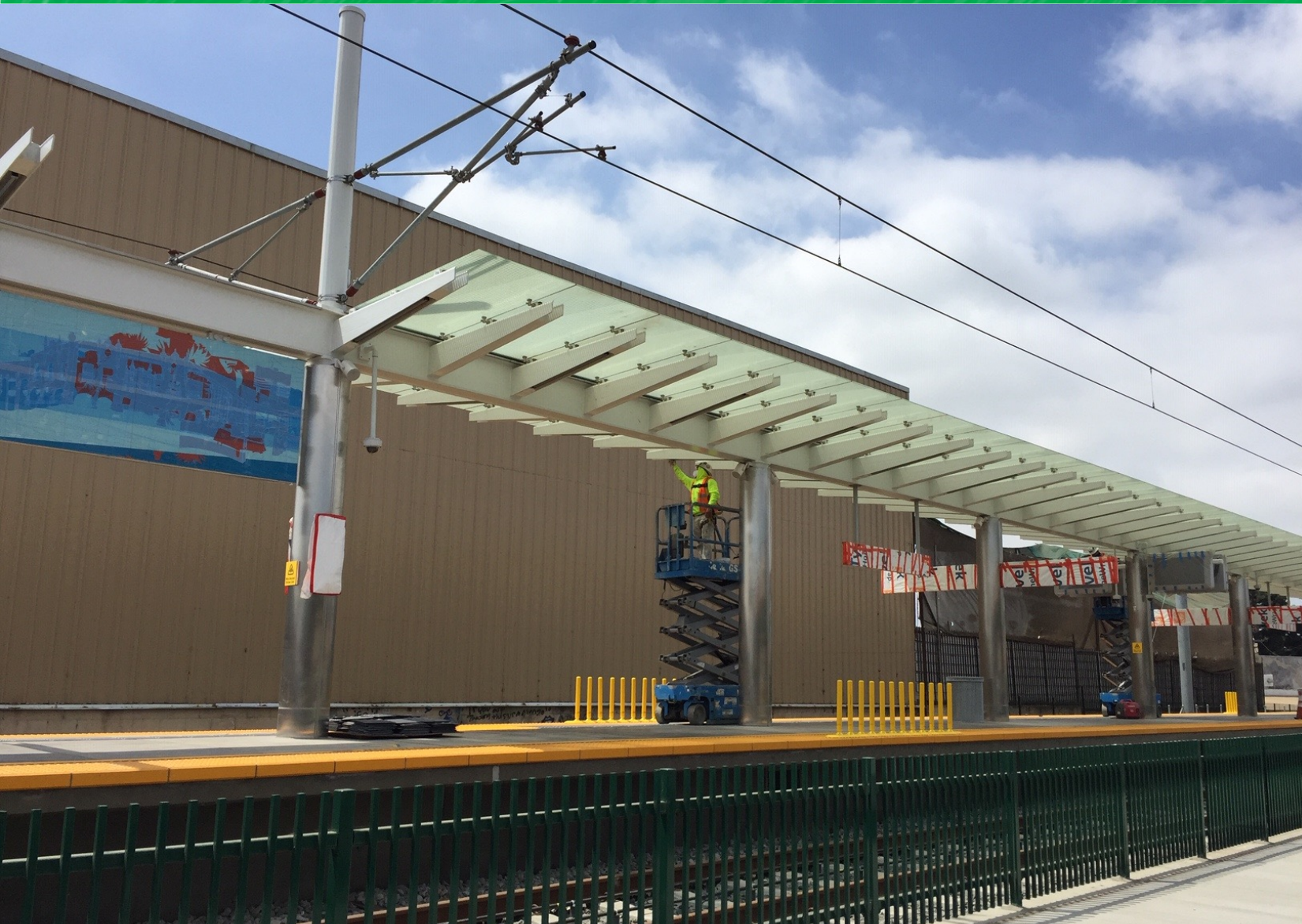
Contractor performing stainless steel cladding
