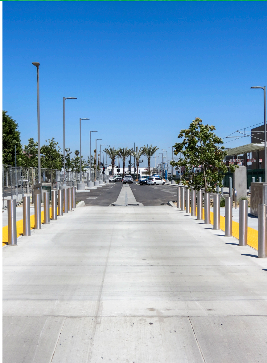
Pedestrian crosswalk, steel bollards, TVM canopy structure
