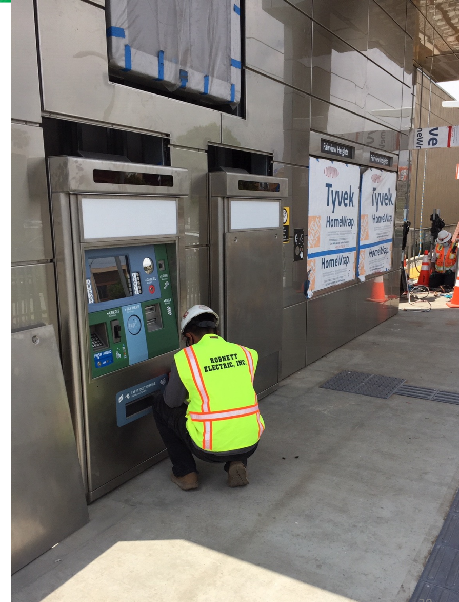
Installing ticket vending machines
