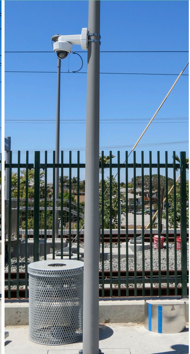
Newly installed CCTV and ETEL with blue light station
