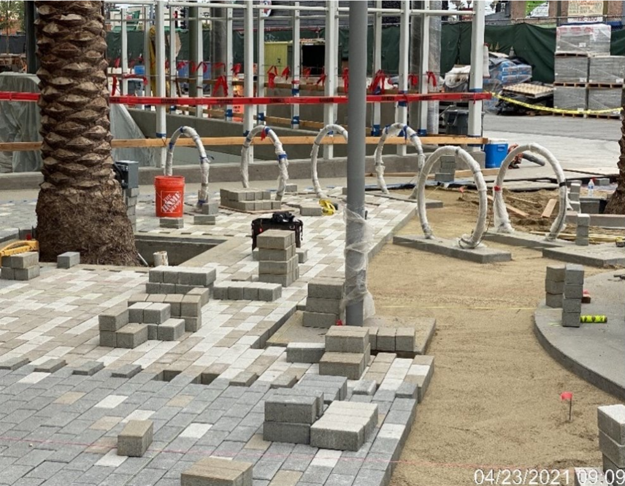
Brick paver installation at MLK Jr Station plaza
