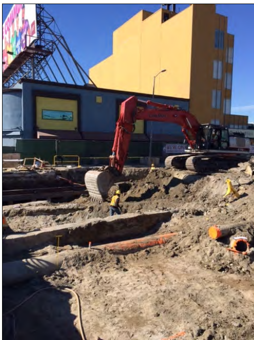
Figure 2-21: Example of In-Street Excavation
