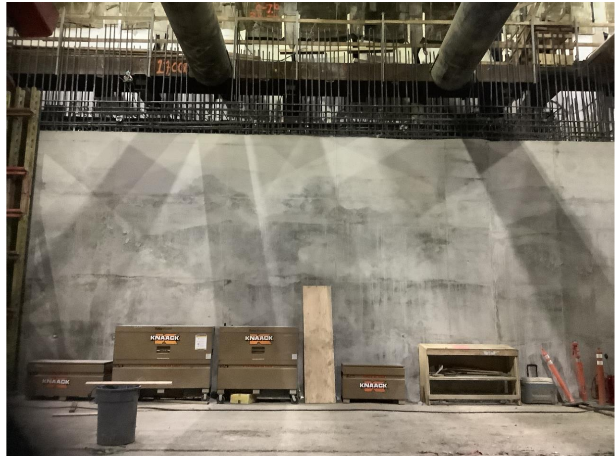
Progress of installing exterior walls.
