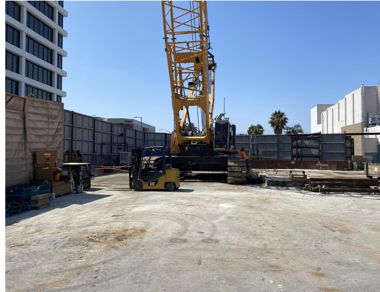
Location of TBM load out
