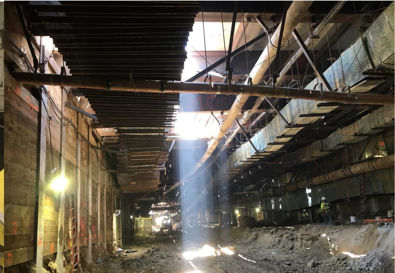
A look inside station excavation in Century City
