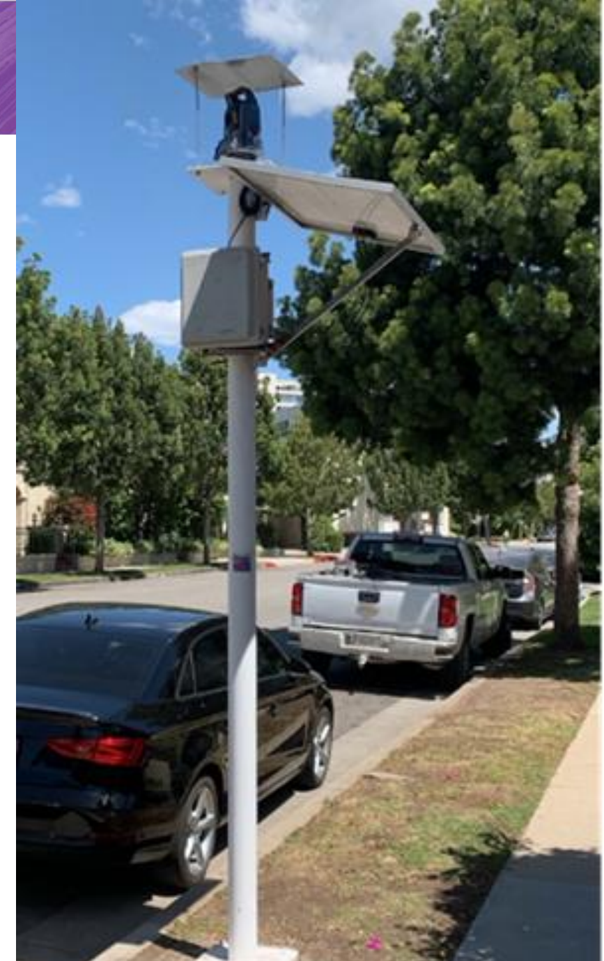
Example of 10-foot geotechnical instrumentation pole.
