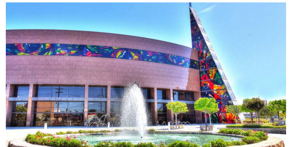
The West Angeles Cathedral is a major destination adjacent to the station.
