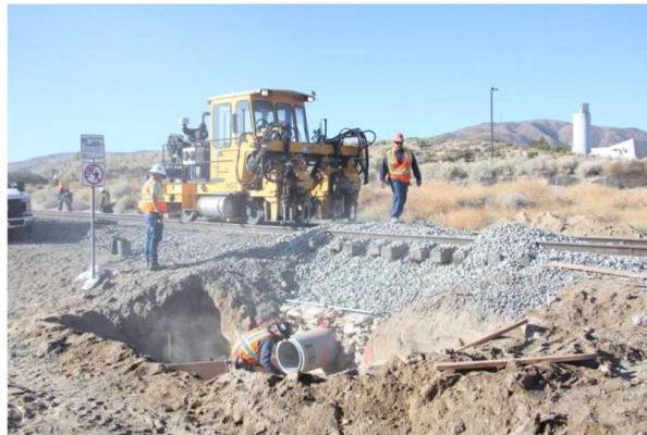
Culvert Replacement at AVL MP 66 Source: Metro (WSP)
