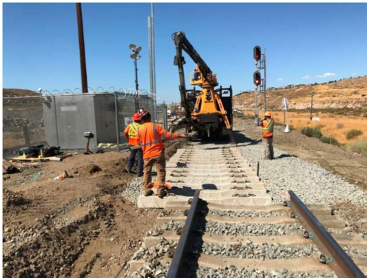
Track Replacement at CP Soledad Source: Metro (WSP)
