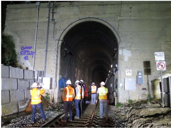
Tunnel 25 – Source: Metro (WSP)
