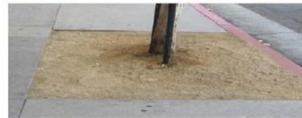
Tree Well 4' x 6' decomposed granite tree well (on blocks without existing tree grates)
