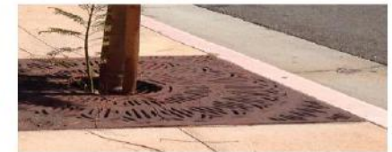
Tree Grate 4' x 4' iron tree grate to match existing (on blocks with existing tree grates)
