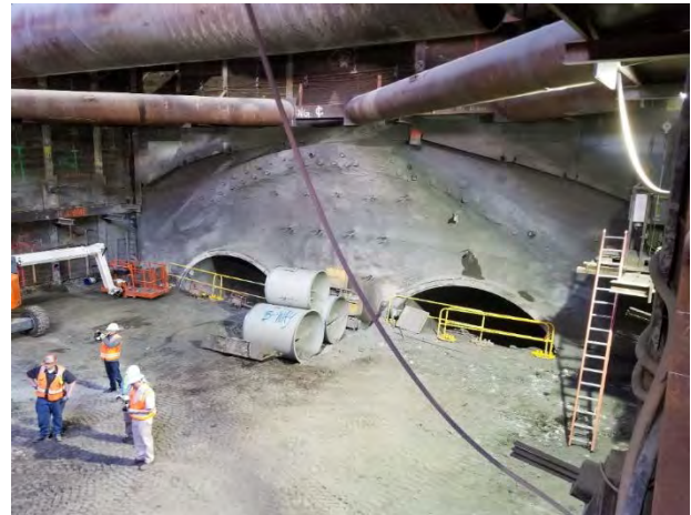
Face of SEM Cavern at Historic Broadway Station
