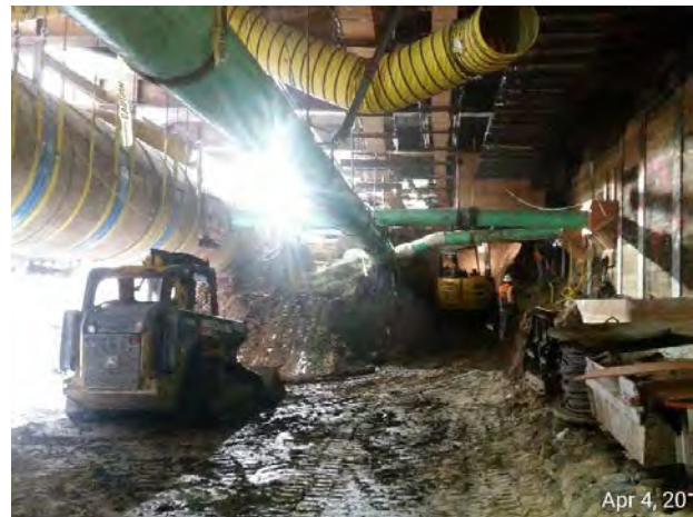
Excavation near South Access Shaft at 5th/Flower
