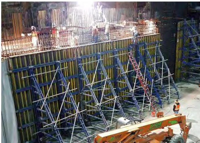
Wall forms for concrete placement at Grand Av Arts/Bunker Hill Station
