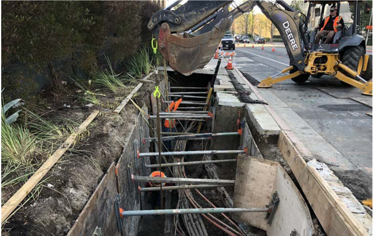
AT&T Utility Work in Century City
