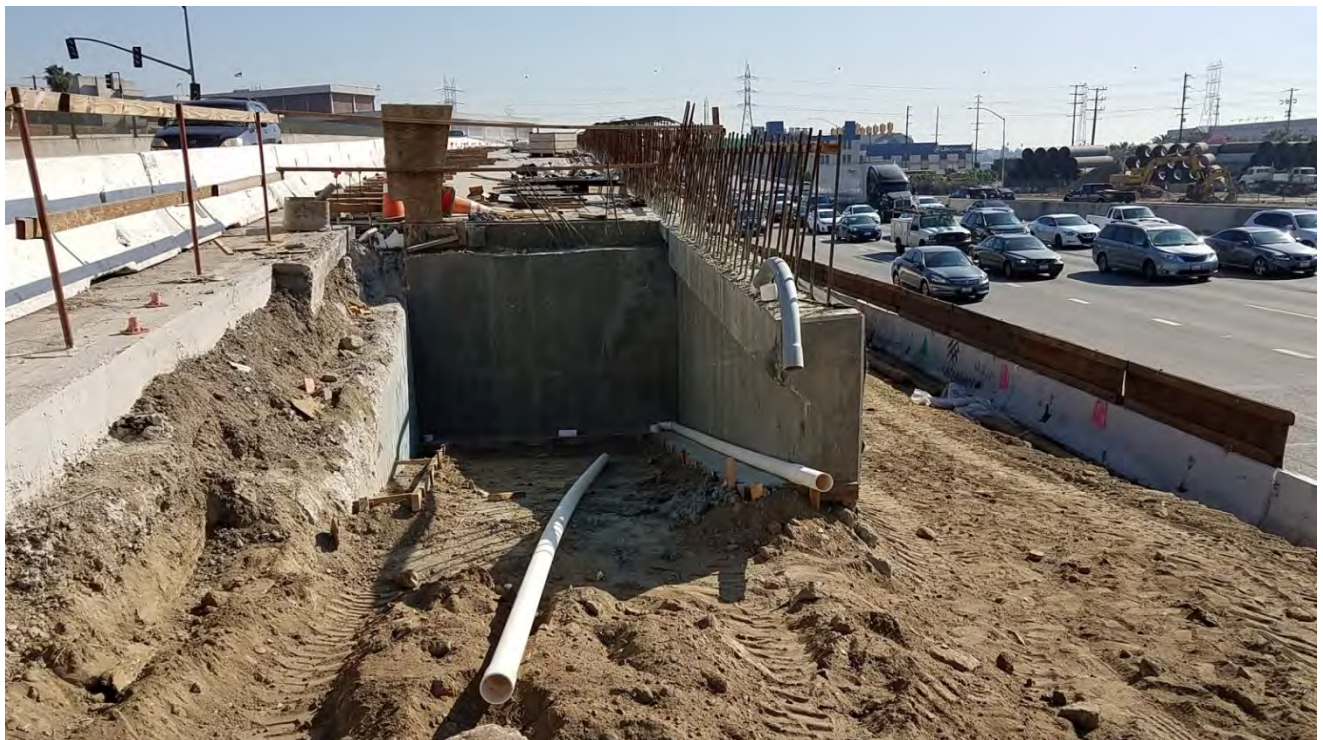
Drain at Abutment 1.
