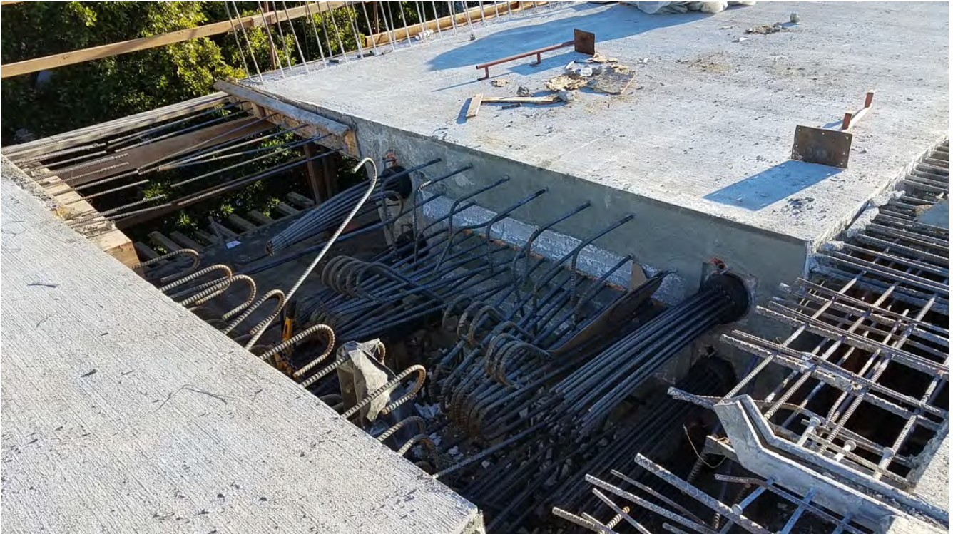
Post Tensioning Frame 4 Left.
