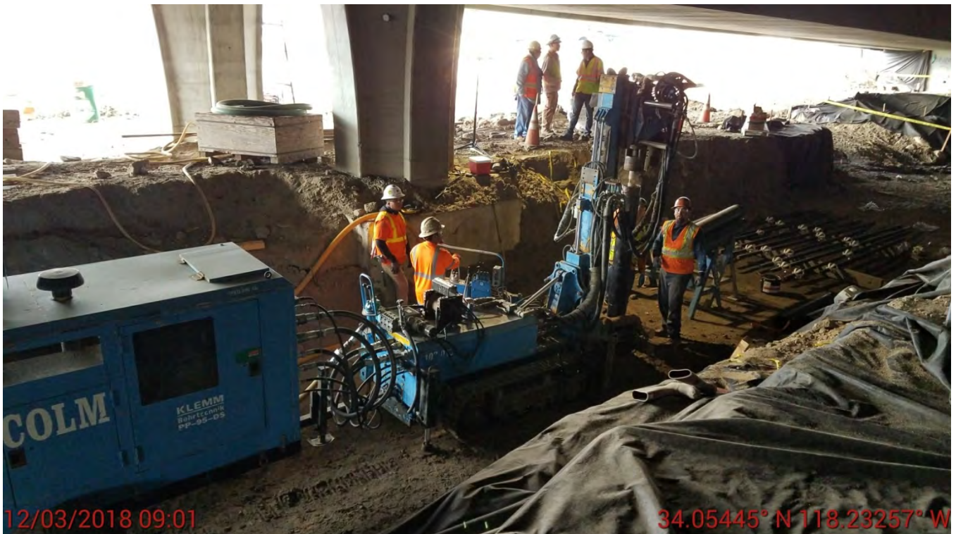
Drill for Micropile Test.
