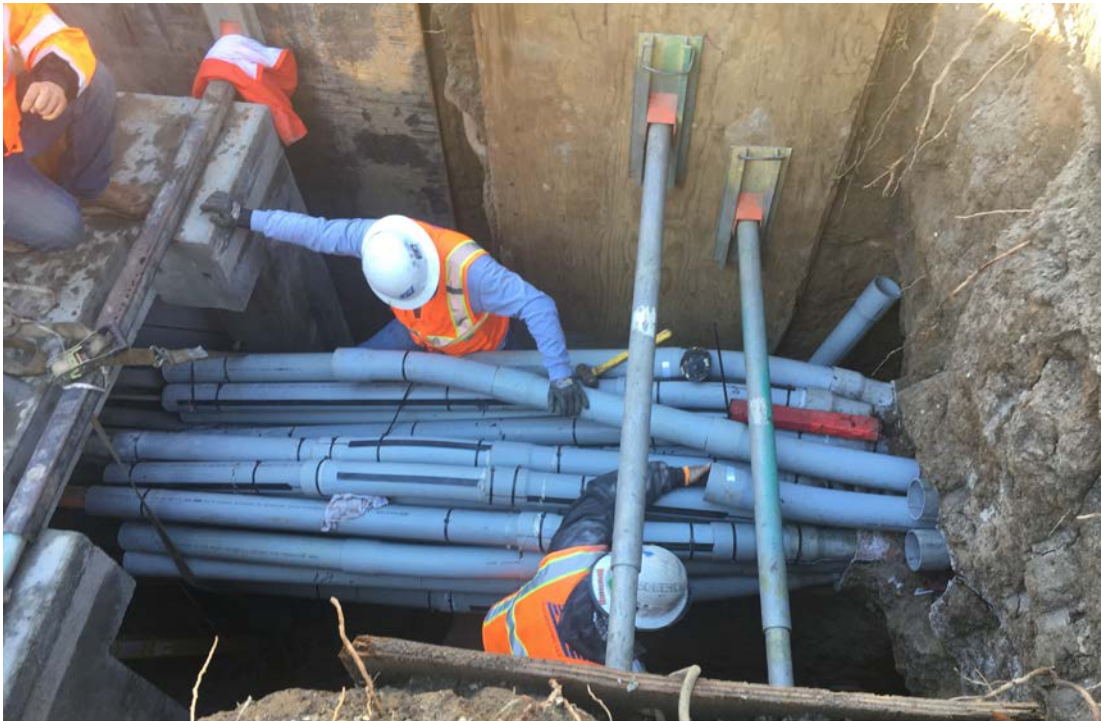
AT&T Conduit Installation in Century City
