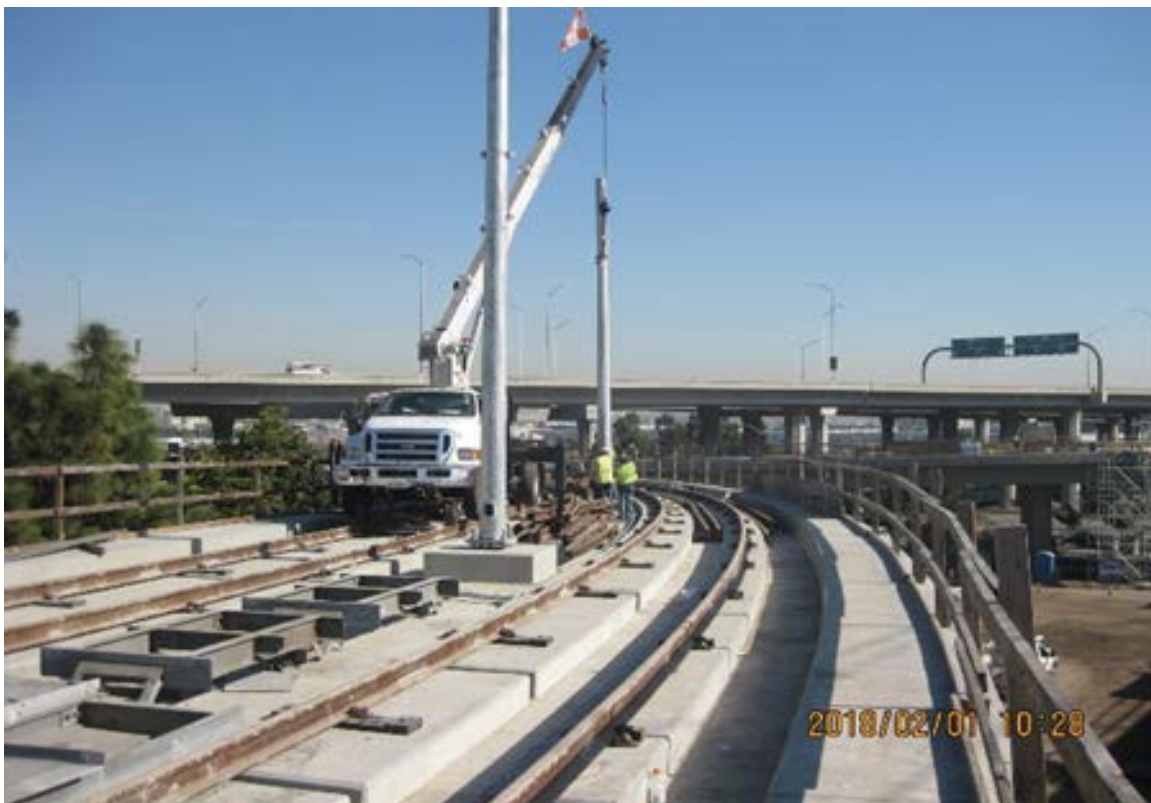
Setting overhead catenary system poles – south end.
