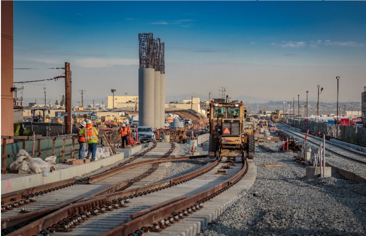
Trackwork at 96 th
