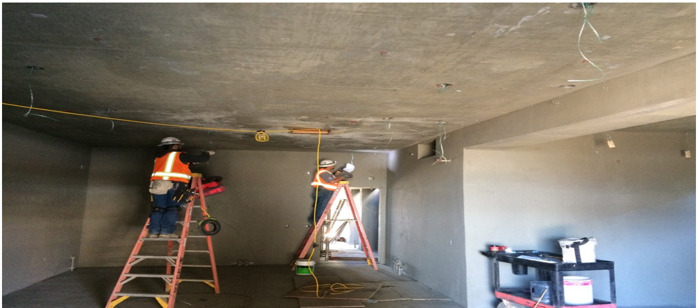
Aviation/Century Bridge – Pulling string and labeling conduit in the service building TC&C.
