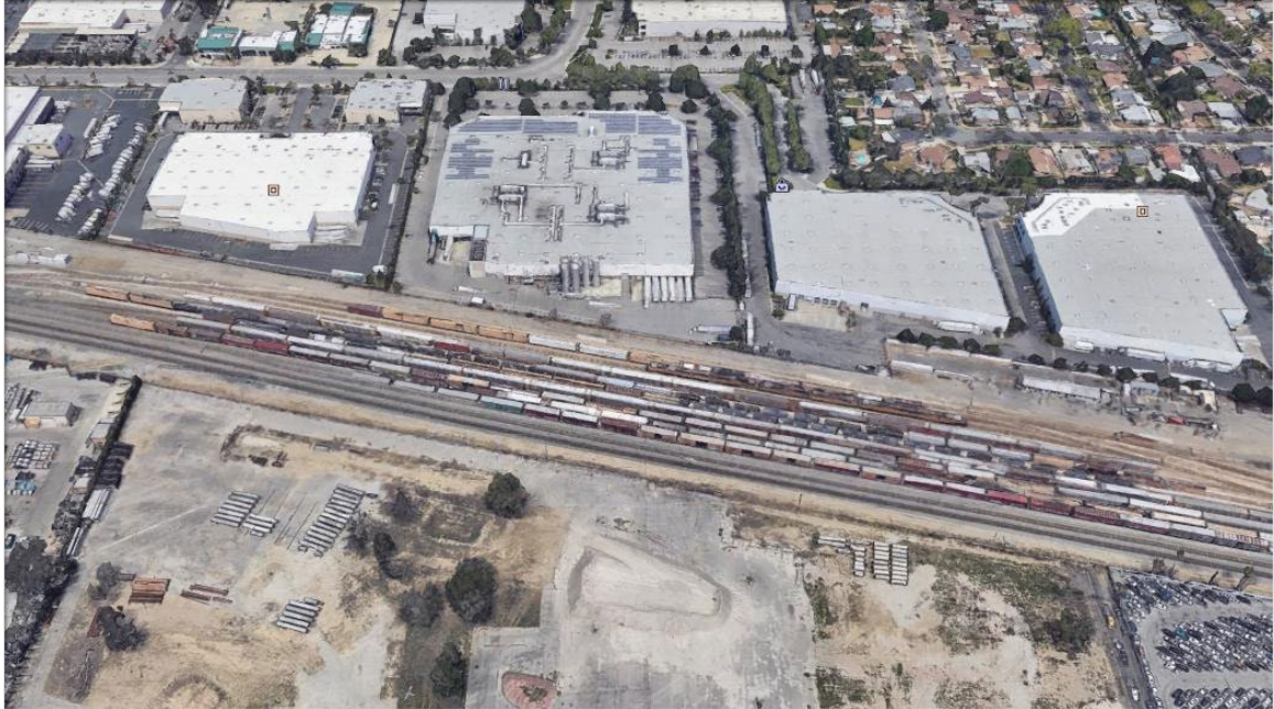
Figure 2-6: UP’s Gemco Yard, MP 455.5 on Ventura Subdivision
