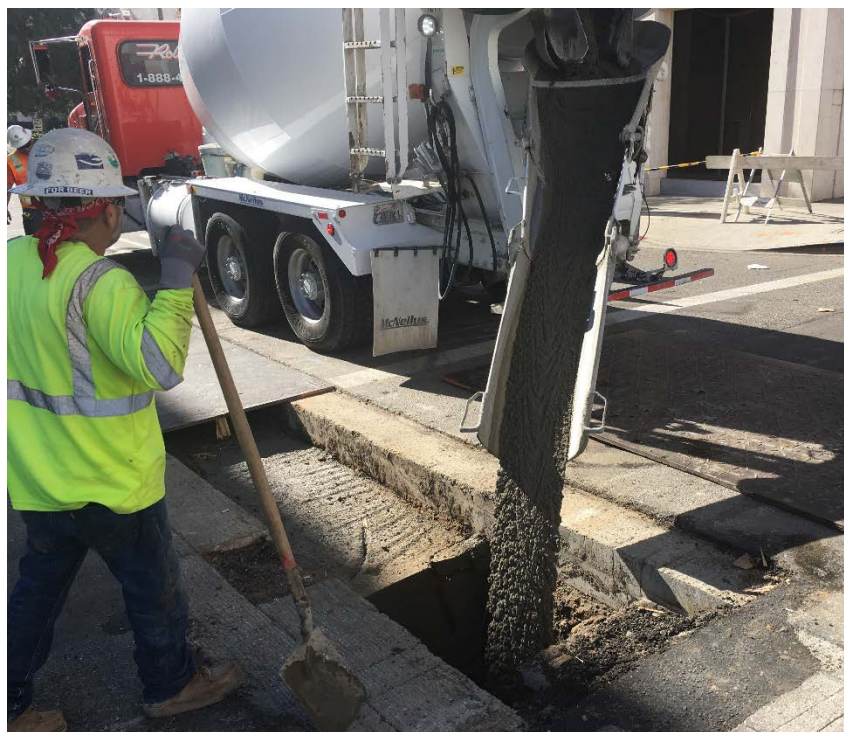
SCE Utility Relocation Work in Beverly Hills
