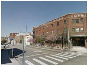
C Looking West
