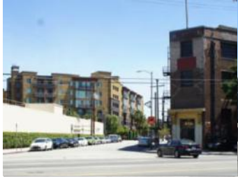
A Looking East
