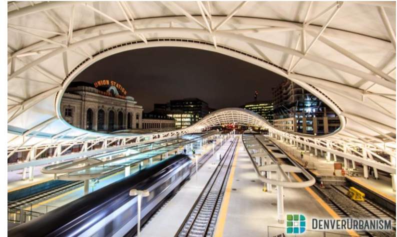
Denver Union Station Transit Center Rail Platforms
