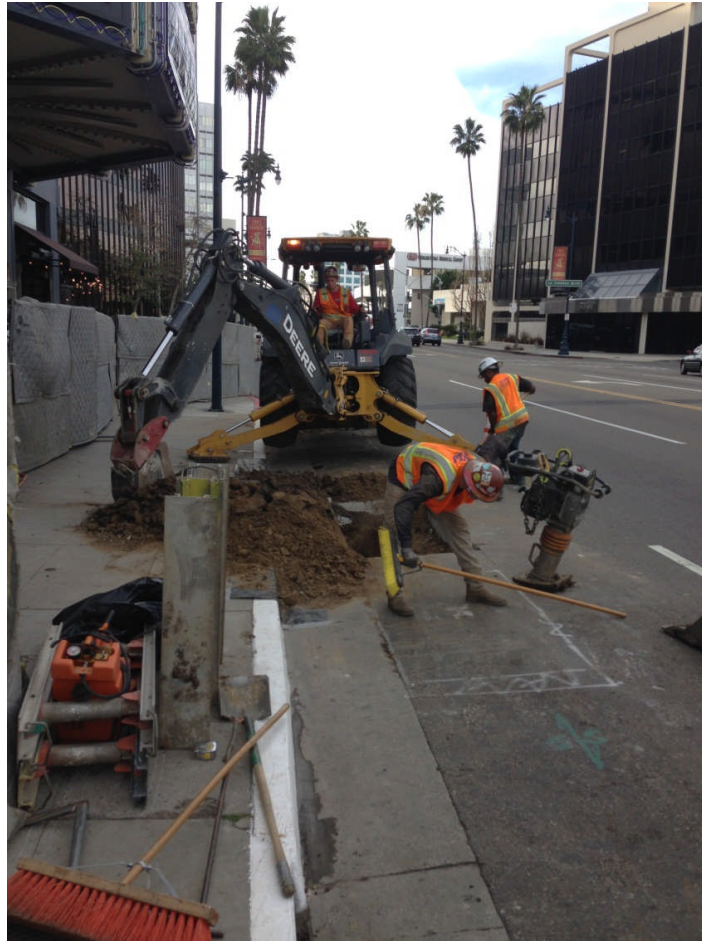
Utility Potholing by VCI at Wilshire/La Cienega
