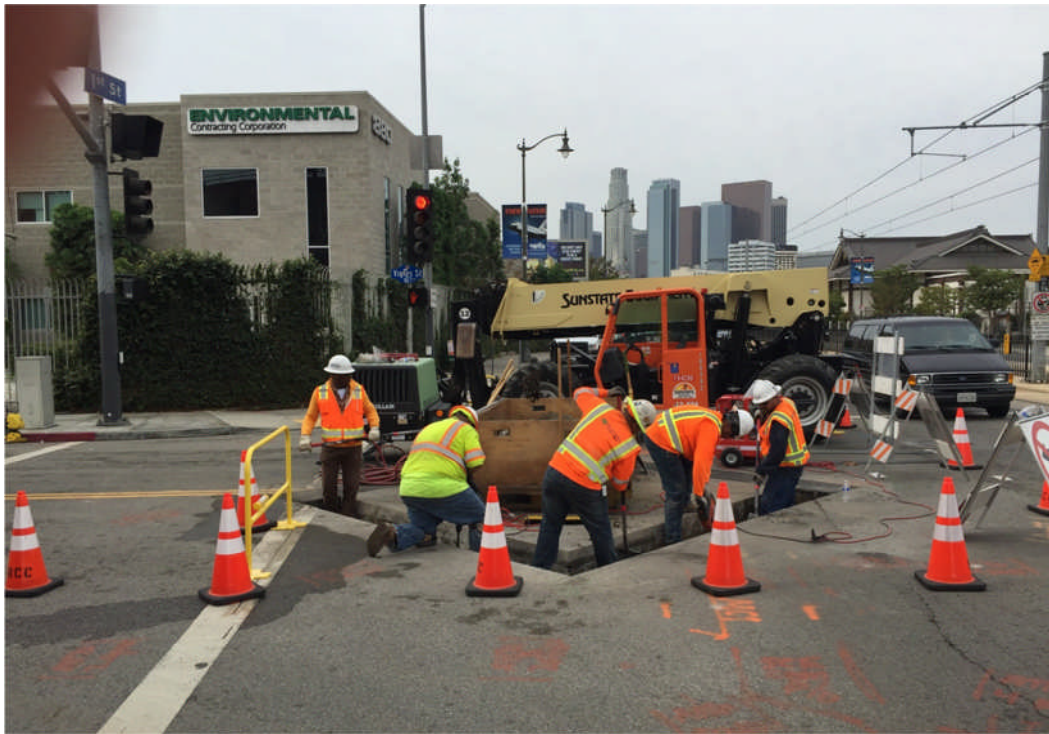
C0980 Contract – Potholing along 1 st Street
