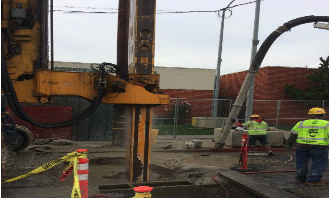
Expo North Headwall Drilling CSM Panel N1.
