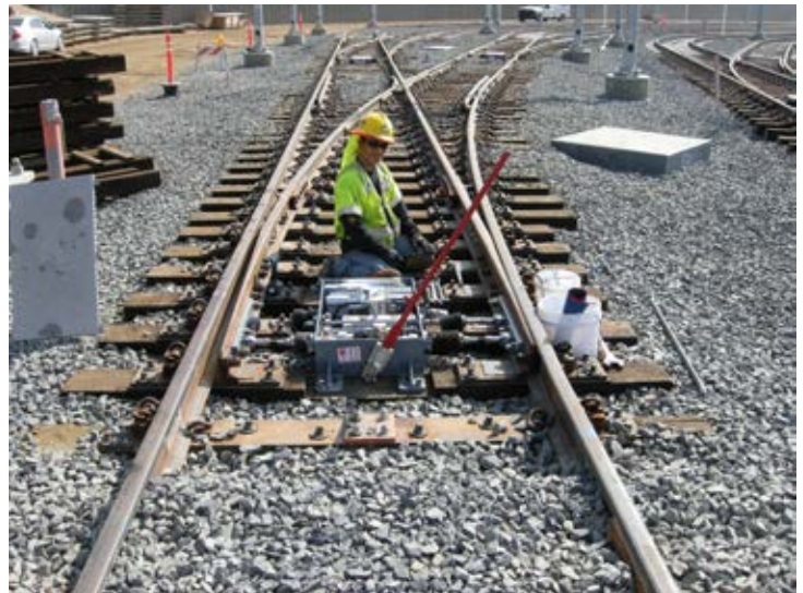
Operations Campus: Track Switch Installation
