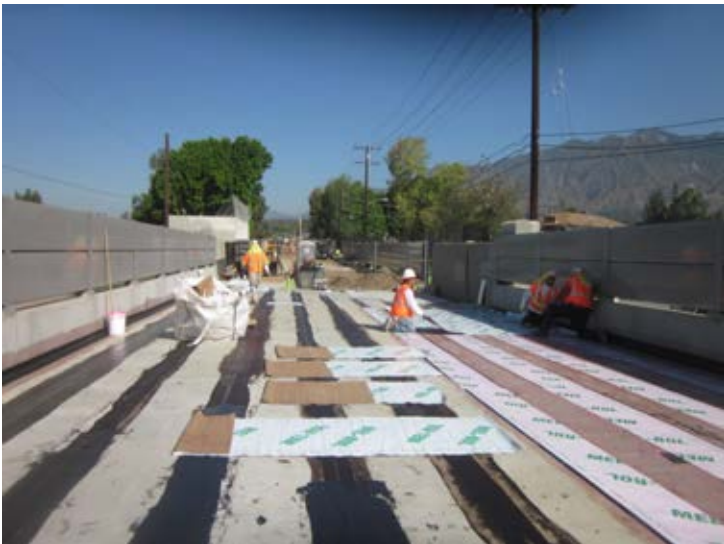
Segment 2: Colorado Bridge Waterproofing
