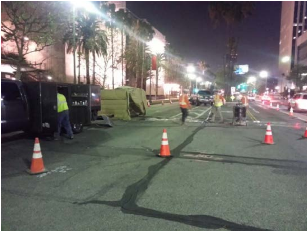
Saw-cutting Pavement using a Noise Blanket Cart near the Wilshire/Fairfax Intersection in Advance of Relocating Utilities
