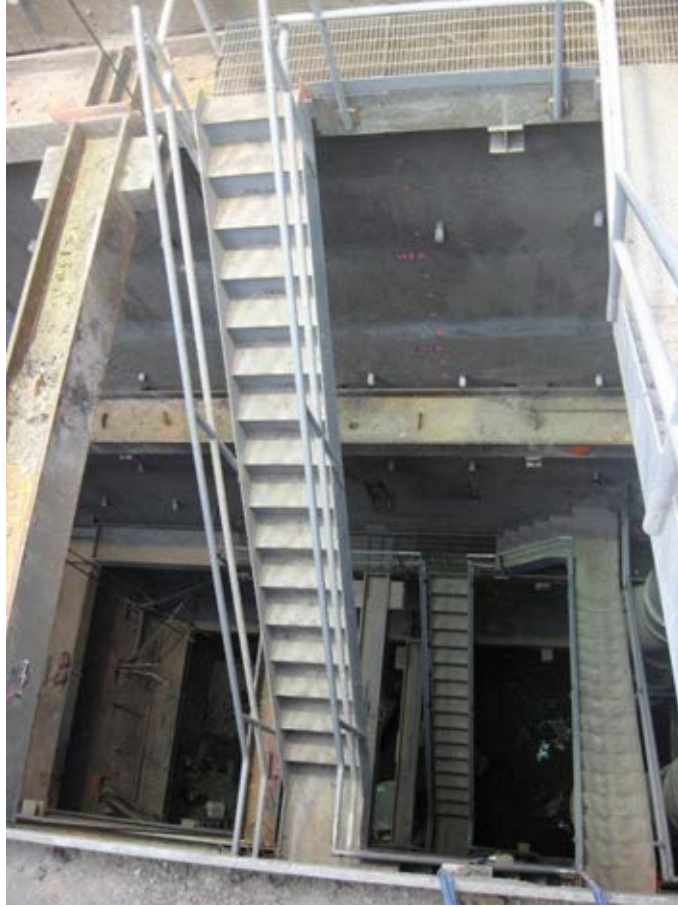
Aboveground View of the Exploratory Shaft
