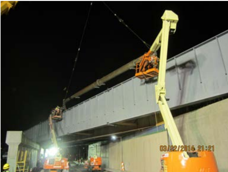
Segment 4: Foothill Bridge - Steel Girder Erection
