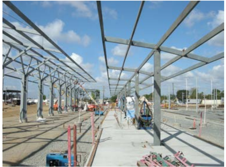
Operations Campus: Progress on Car Cleaning Platform Canopy steel
