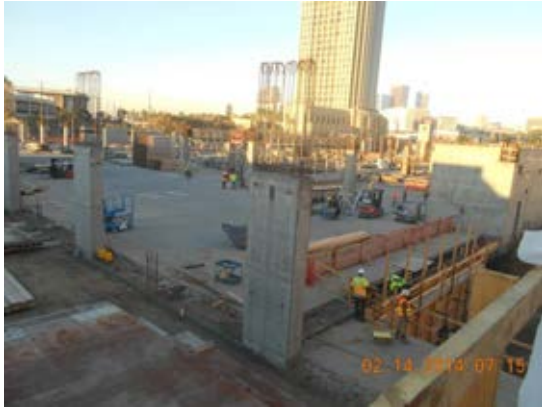
South west view of 1 st level deck at Garage Building.
