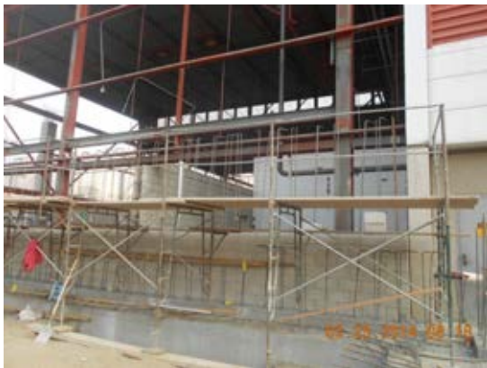
Placement of 1 st lift exterior CMU wall at Old Radiator Shop.
