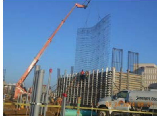
Placement of vertical steel rebar at south walls Area 8.
