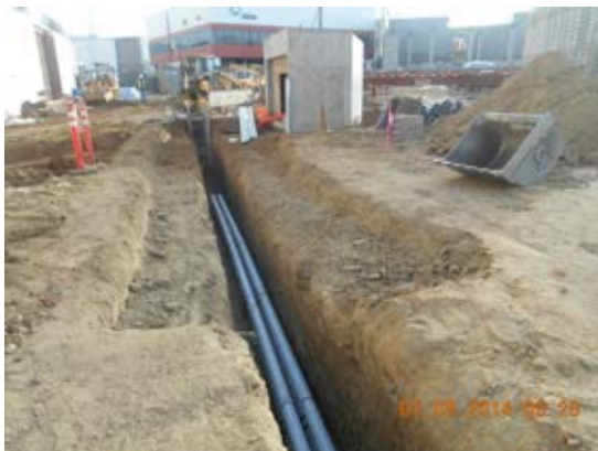
Placement of UG conduits for fiber optic at Metro Driveway.
