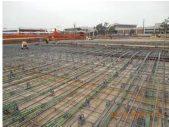
Placement of reinforcement steel at Upper Level Dk Area 7.
