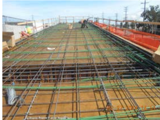
Installation of PT tendons at elevated ramp deck Area 5.
