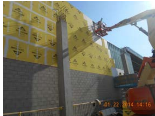
Placement of exterior gyp board at 3hr. wall along Bldg. 1.
