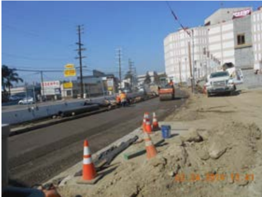
Compaction of subgrade and base at Vignes Street.
