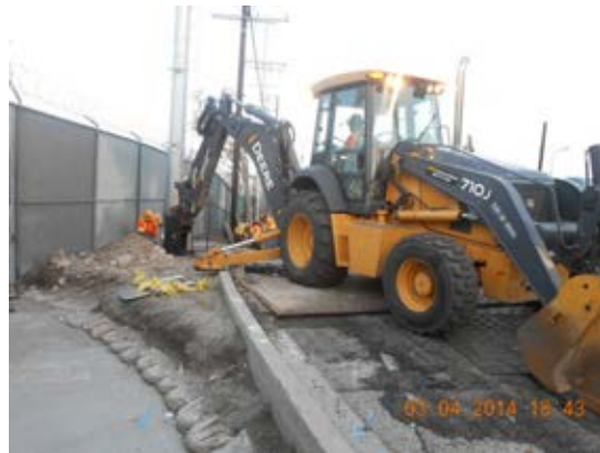
Excavation of UG conduits for DWP stub ups.
