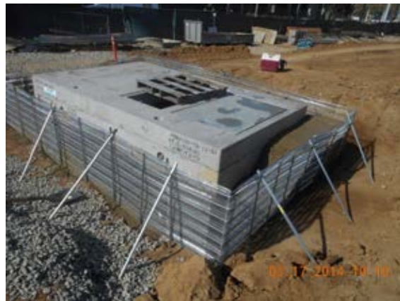
Placement of utility vault at DWP Utility Yard.
