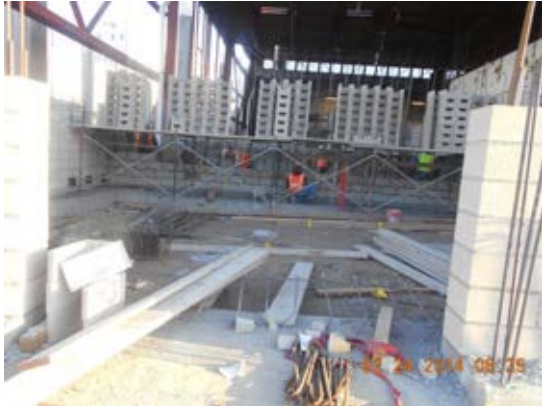
Placement of interior CMU walls at Old Radiator Shop.
