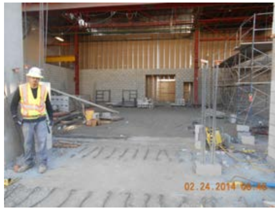
View of interior CMU wall at Old Radiator Shop.
