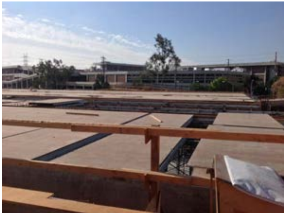
Setting of panel deck forms for roof level at Building B.
