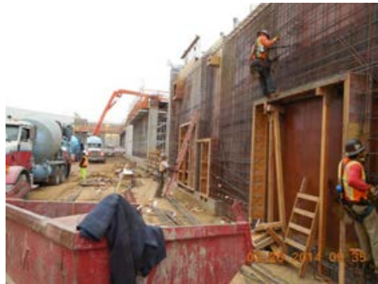
Placement of vertical reinforcement on walls at Bldg. B North.
