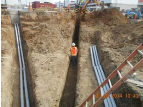
Installation UG conduits to DWP Utility Yrd from Cesar Chavez.
