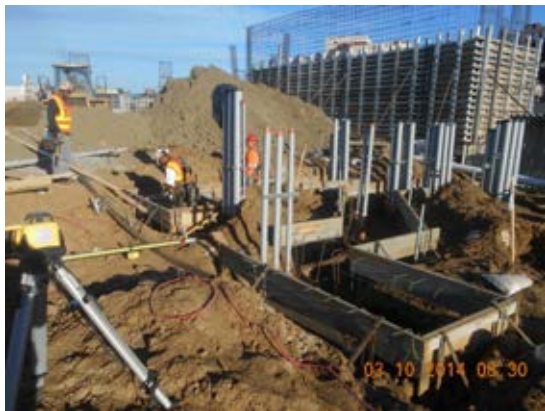
Concrete formwork for UG conduits at DWP Utility Yard.
