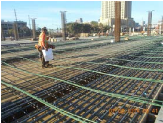
Steel rebar and tendons placement 1 st level deck at Area 6.
