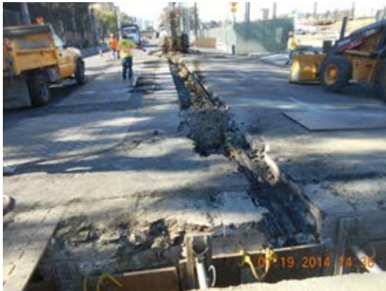
Excavation of trenching for UG utilities along Cesar Chavez.
