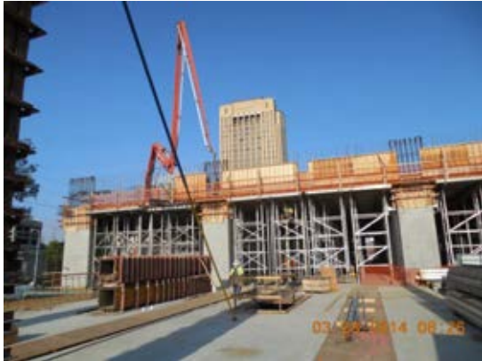
Concrete placement at Roof Deck No. 14.
