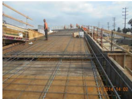
Placement of steel rebar at ramp deck panel for pour #4.
