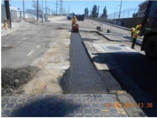
AC patching of UG utilities trench at Cesar Chavez.
