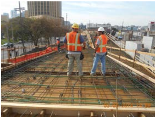
Placement of steel rebar and PT cables at Ramp in Area 5.
