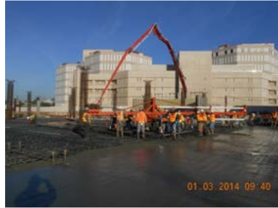
Placement of concrete pour #3 at elevated deck Area 7.
