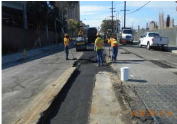
AC patch of UG trenching along Cesar Chavez.
