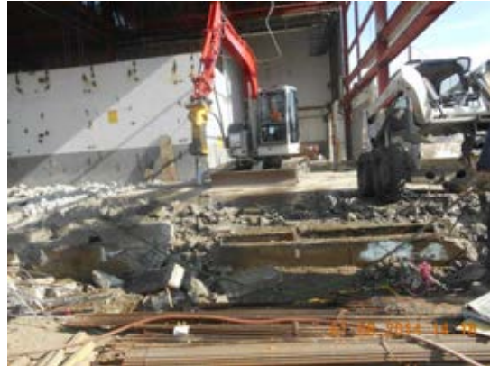
Demolition of existing interior SOG at old Radiator Shop.
