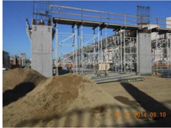
Placement of upper level deck panels and formwork.
