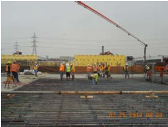
Concrete placement at Upper Level Building B Area 7.
