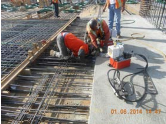
Stressing of post tendons cables at Area 5.
