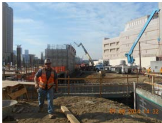
Lifting and setting of UG vault at Metro Driveway.
