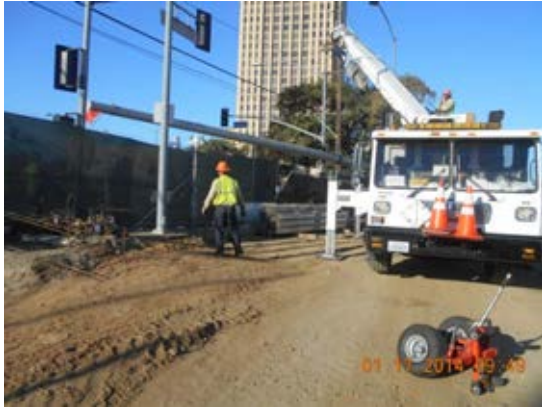
Installation of electrical poles by DWP along Cesar Chavez.
