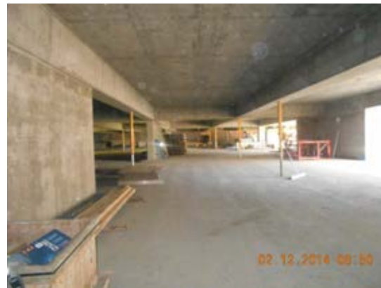
View of underside level deck at Garage Building.
