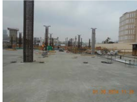
Partial view of 1 st Level concrete deck at Parking Garage.
