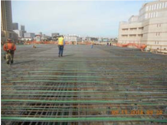
Placement of steel reinforcement at roof level deck Area 7.
