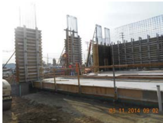
Placement of wall formwork at Maintenance Building.
