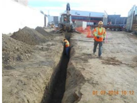
Excavation of UG fiber optic conduits at Metro Driveway.
