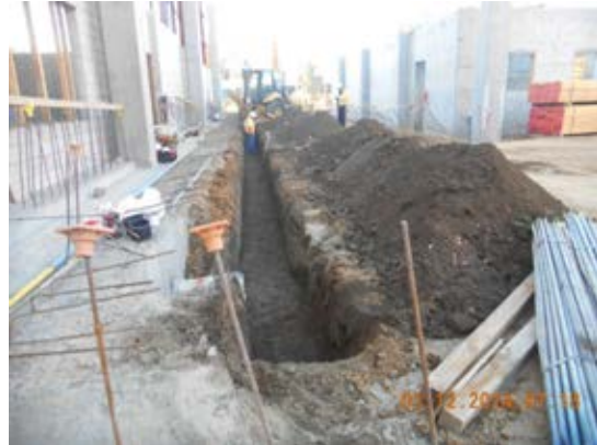
Excavation of footing at Maintenance Building.
