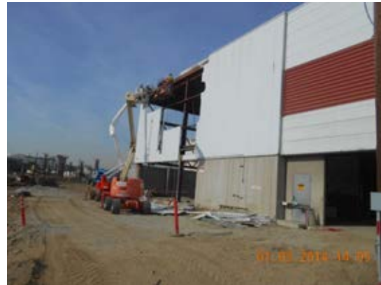
Demolition of exterior walls at old Radiator Shop.
