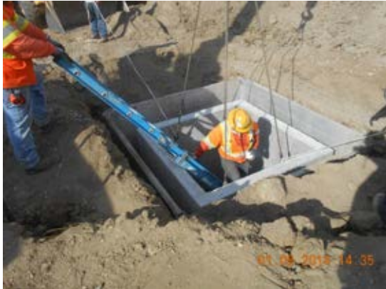
Setting of UG vault at Metro Driveway.
