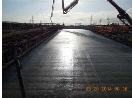
Placement of concrete at Elevated Ramp Deck #3 Bldg. B.
