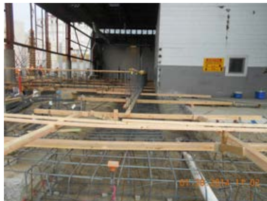
Placement of rebar for footing and foundation at Maint. Bldg.
