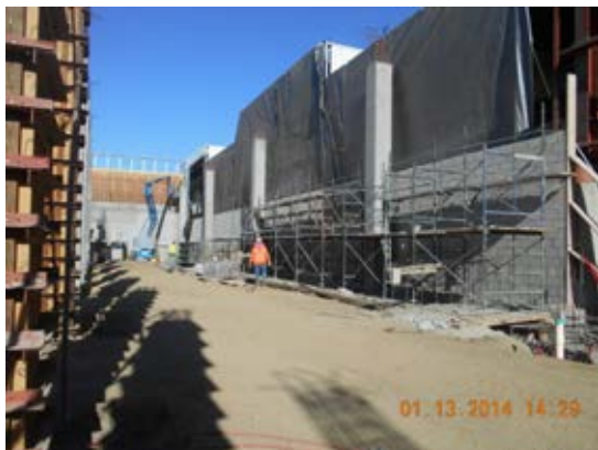
Placement of exterior CMU wall along Building 1.
