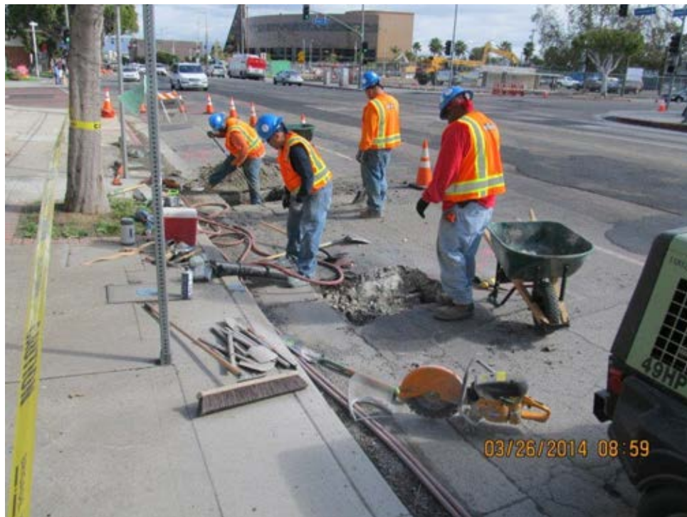
Potholing on Crenshaw Boulevard near Rodeo Street.
