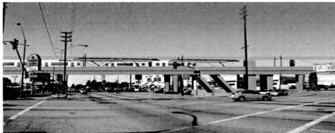
Aerial structure across Manchester Avenue.
