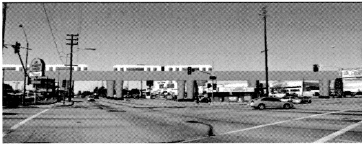
Aerial structure across Manchester Avenue.
