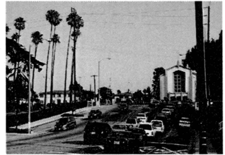
View of Centinela Avenue at Florence Ave/Harbor Subdivision. Traffic movements along with pedestrian flows to a nearby Vincent Park, church and school are major local concerns. The crossing is at the top of a slight incline.
