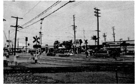
Grade Crossing at Manchester.
