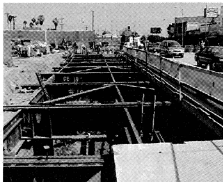
Cut and Cover Construction Goldline Eastside Extension
