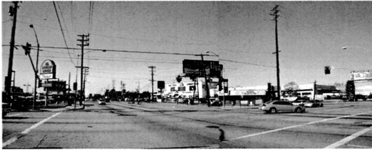
Existing view of the Aviation Boulevard/Manchester Avenue intersection.
