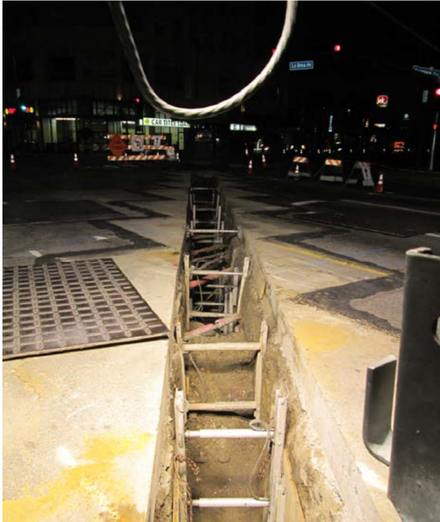
Utility Trench South of Wilshire by the C1048 (Wilshire/La Brea) Contractor
