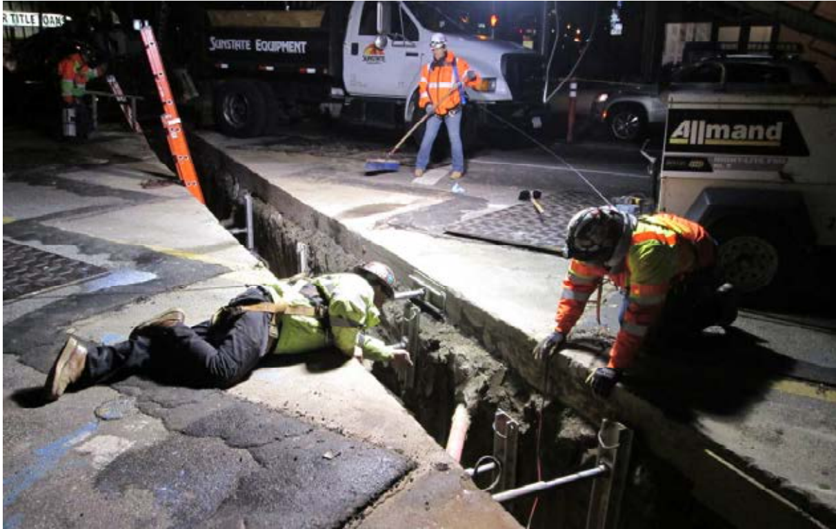
Utility Trenching by the C1048 (Wilshire/La Brea) Contractor
