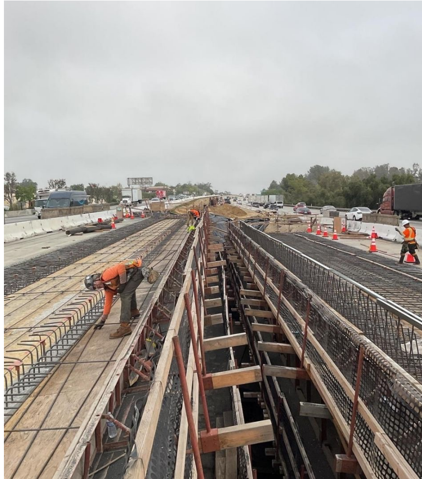
Butte Canyon Bridge, May 2023
