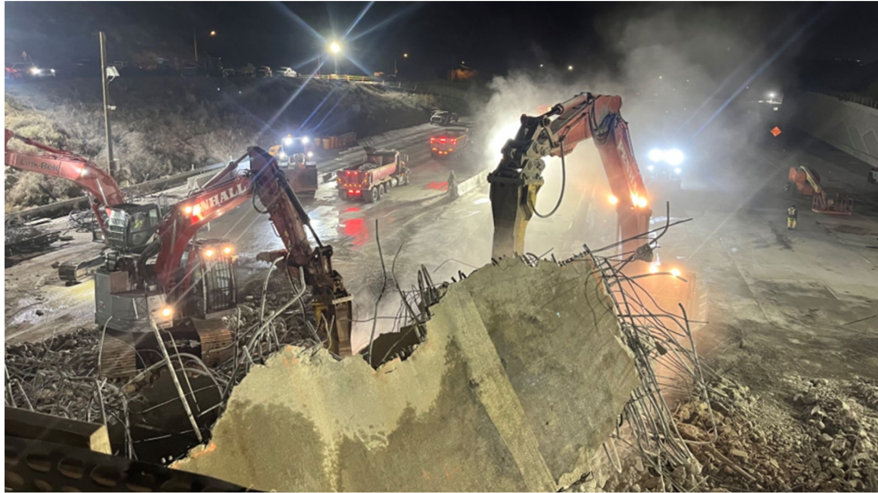
Weldon Canyon Rd Bridge Demolition, November 2023
