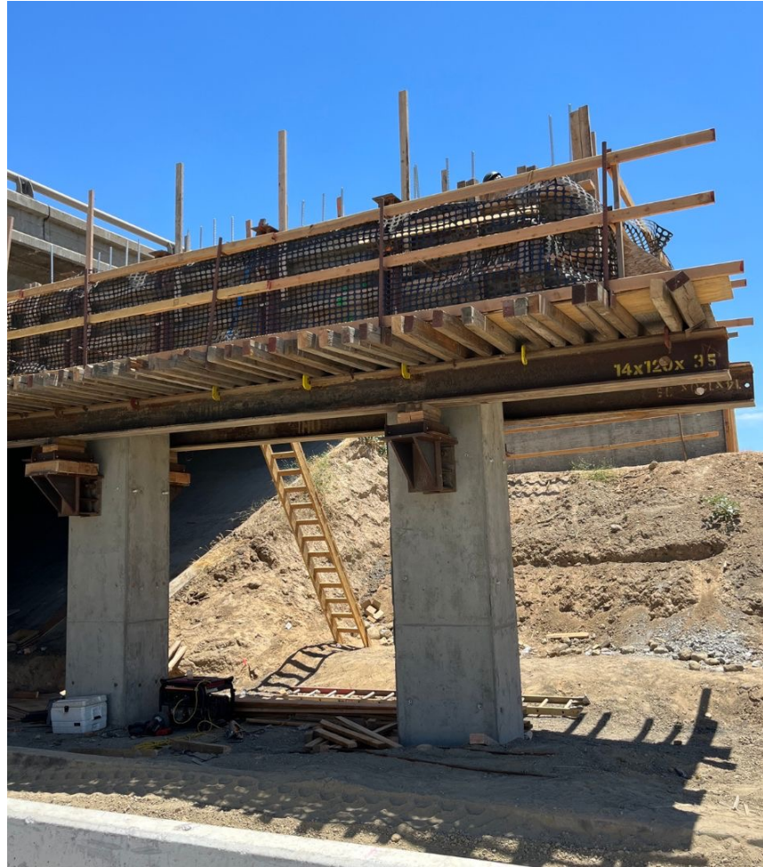
Rye Canyon Rd Bridge, August 2023
