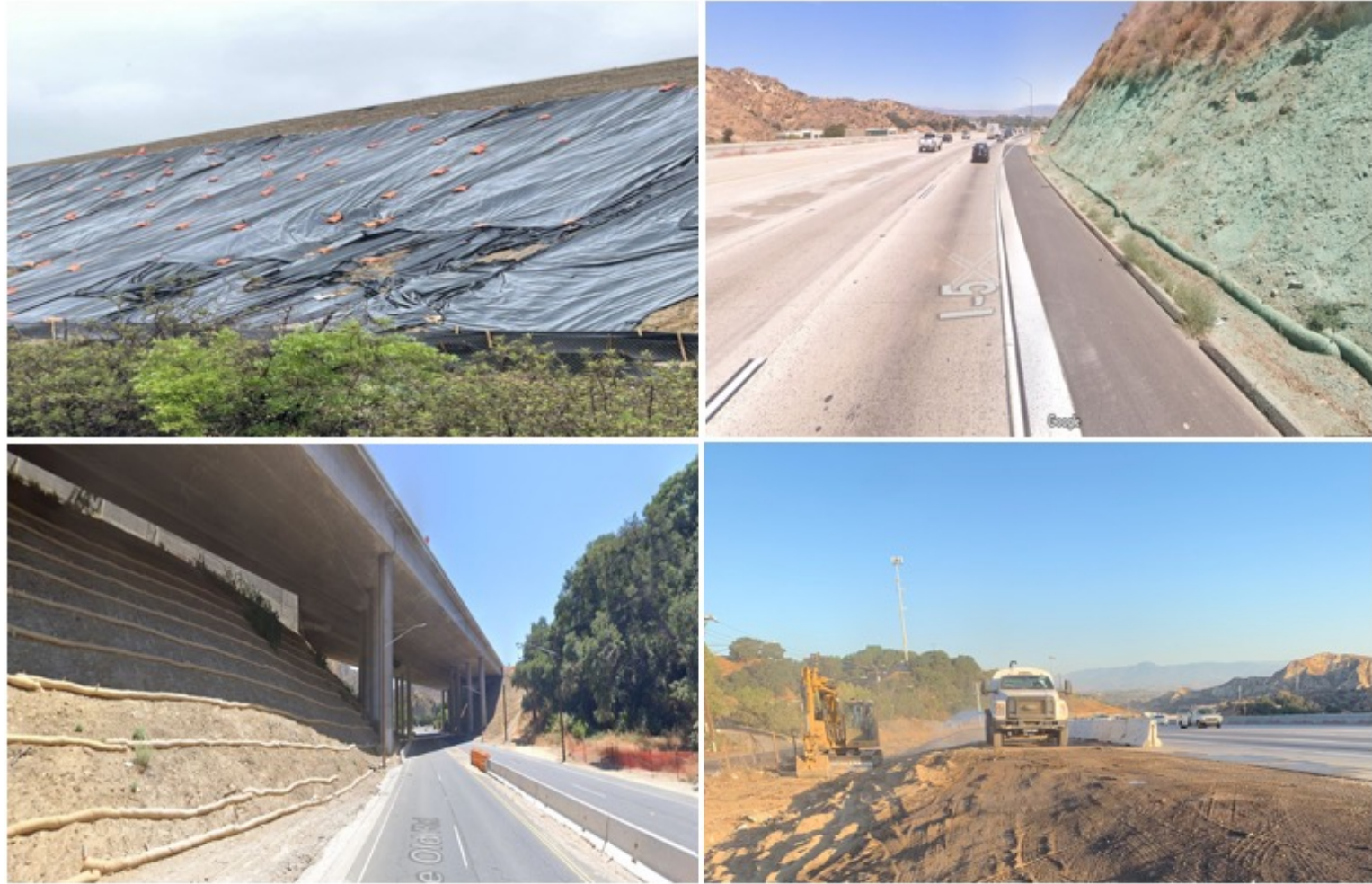
Examples of typical erosion control and dust mitigation methods used on the project
