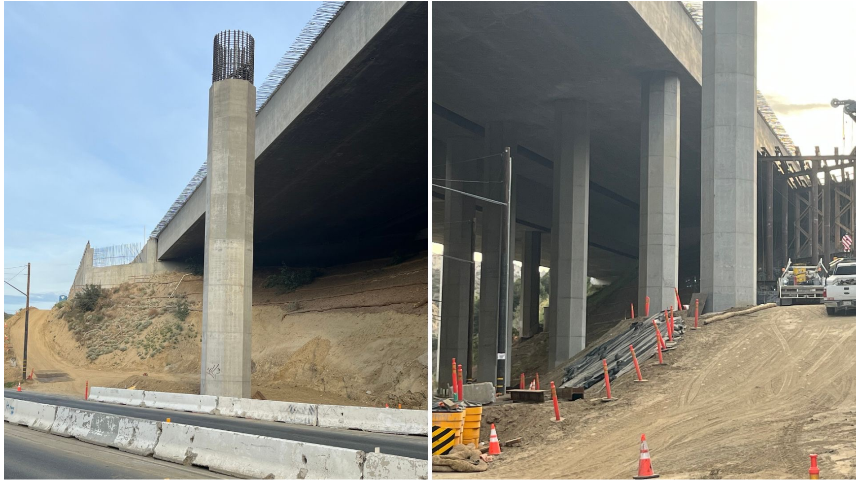
Falsework grading at Gavin Bridge, November 2023
