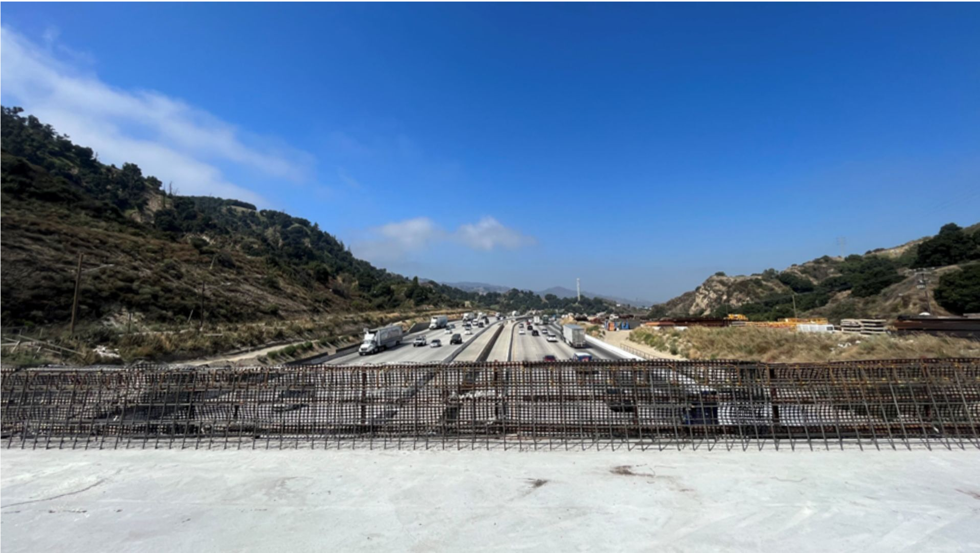
Weldon Canyon Rd bridge barrier installation, November 2023
