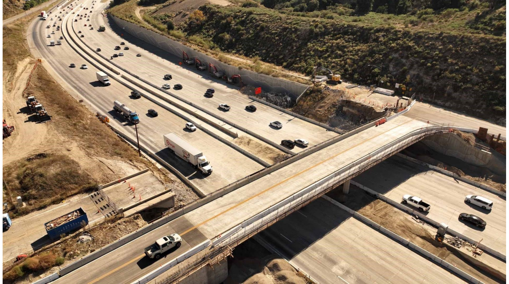
New Weldon Canyon Rd bridge, November 2023
