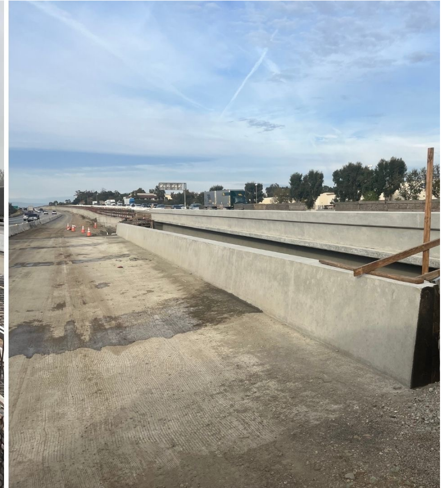
Butte Canyon Bridge, November 2023
