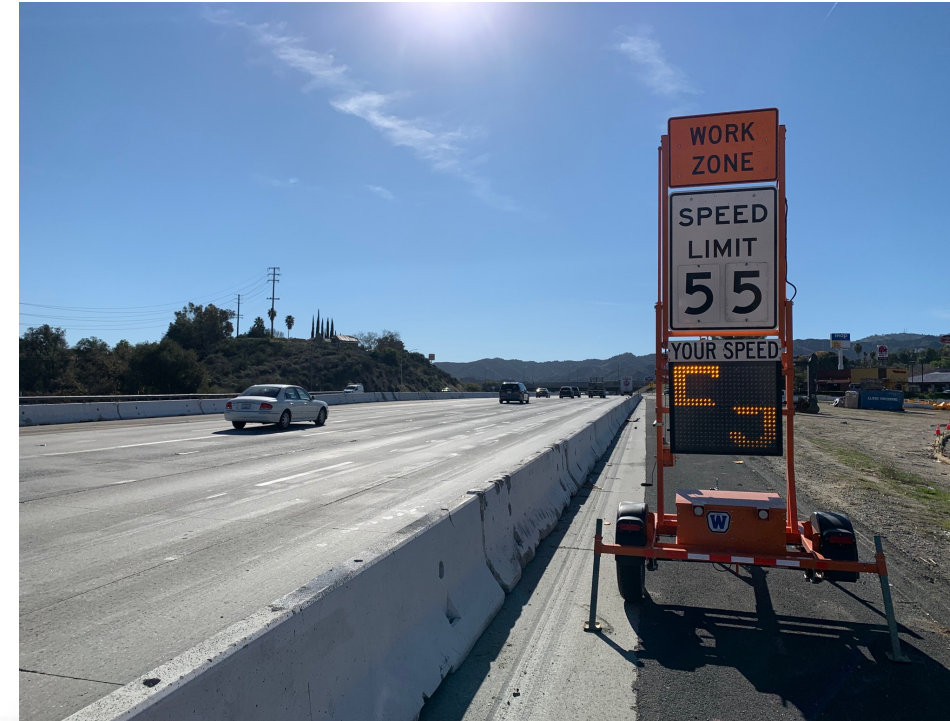
Work zone speed limit signage
