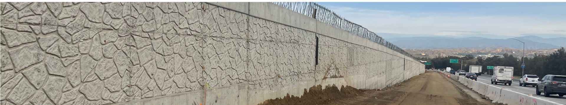
Center median retaining wall backfilling, November 2023
