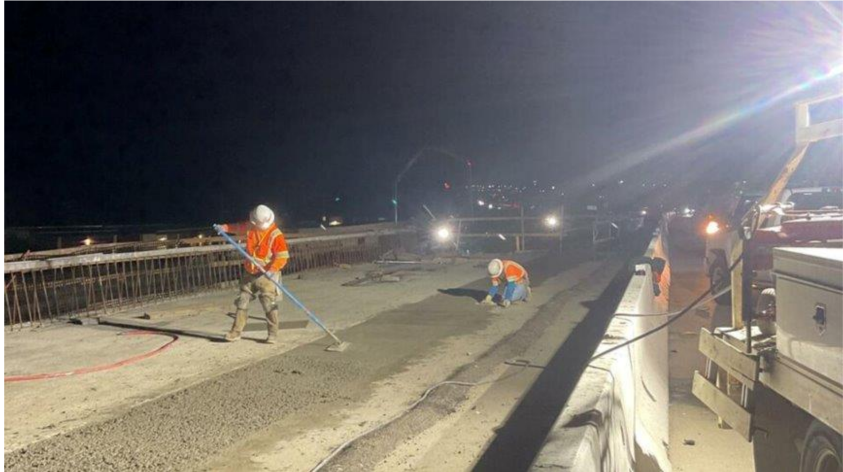
Calgrove BI Bridge concrete setting, June 2024
