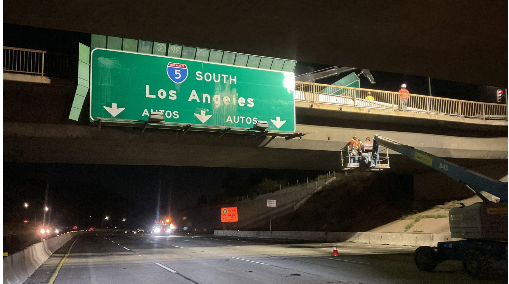
Overhead Sign Removal at Weldon Canyon Rd Bridge – September 2023
