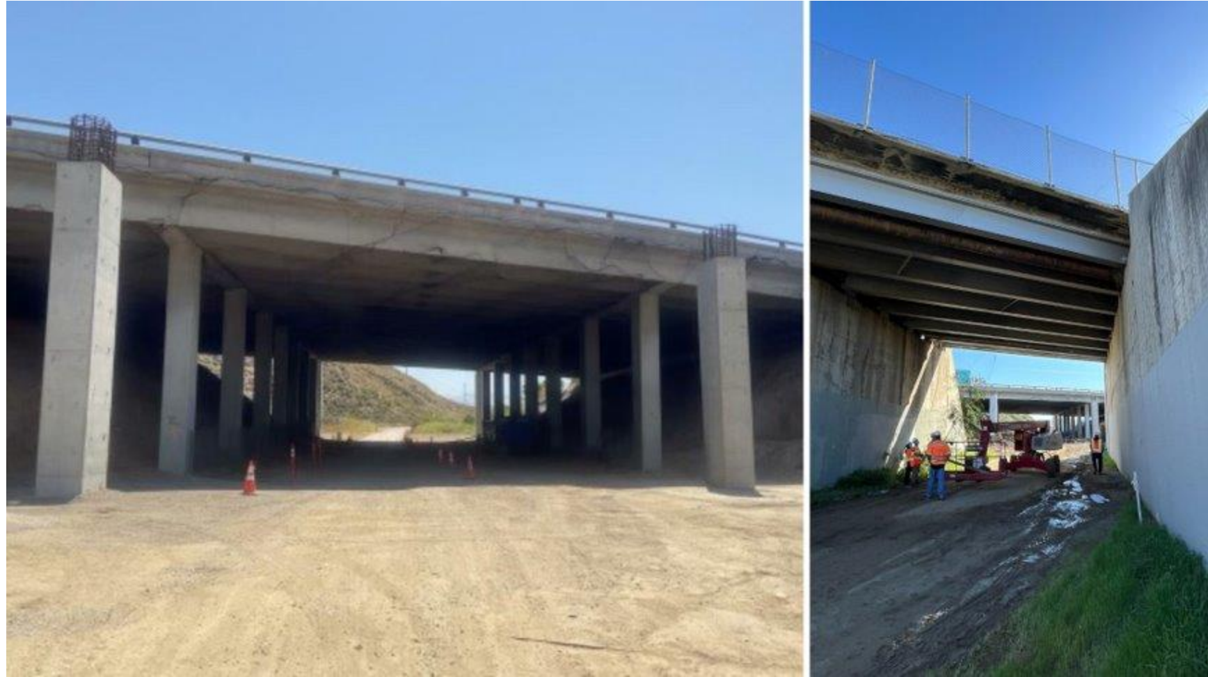
Santa Clara River Overhead Crossing bike path, July 2024
