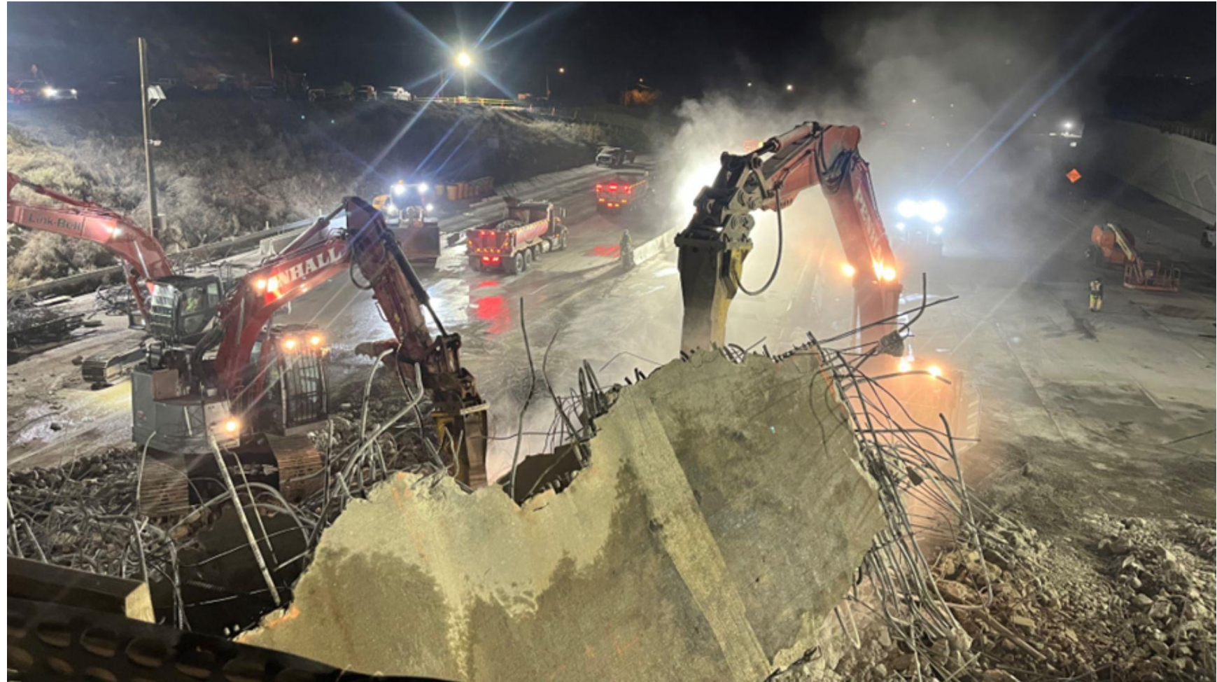
Weldon Canyon Rd Bridge Demolition, November 2023
