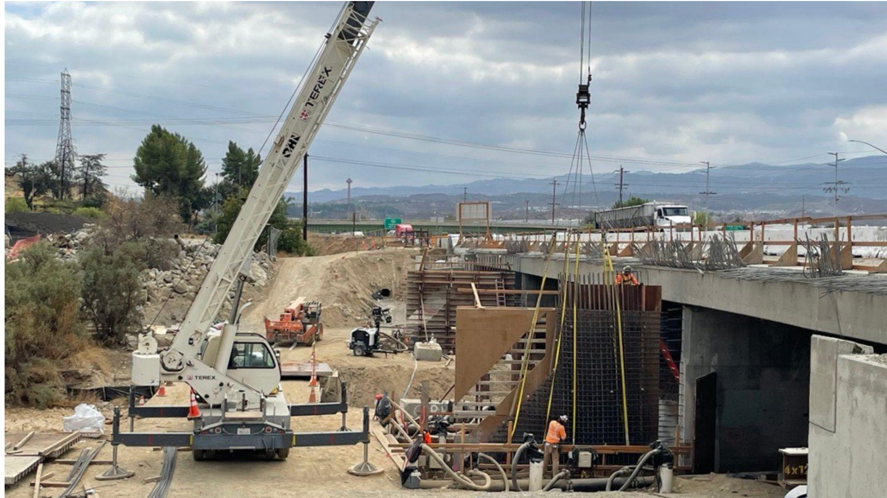
Castaic Creek Bridge, September 2024
