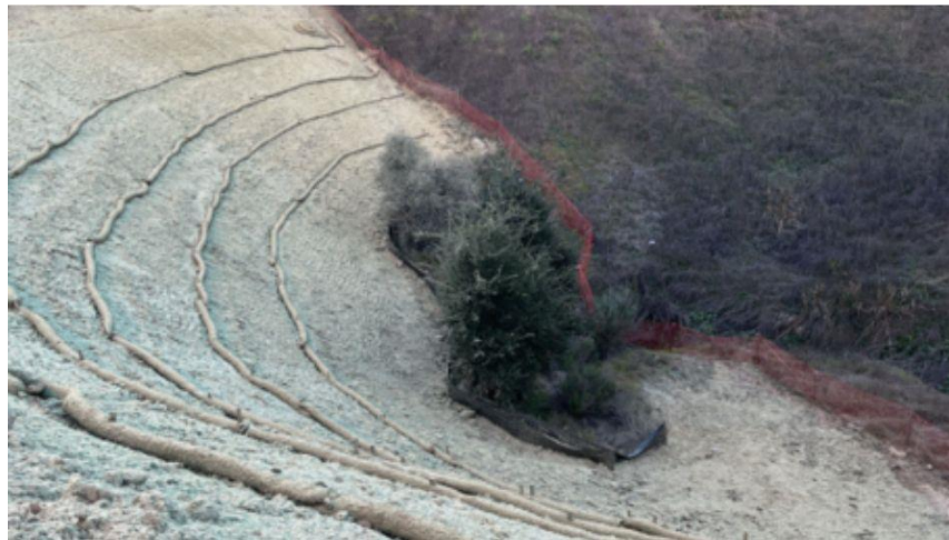
Examples of typical erosion control and dust mitigation methods used on the project
