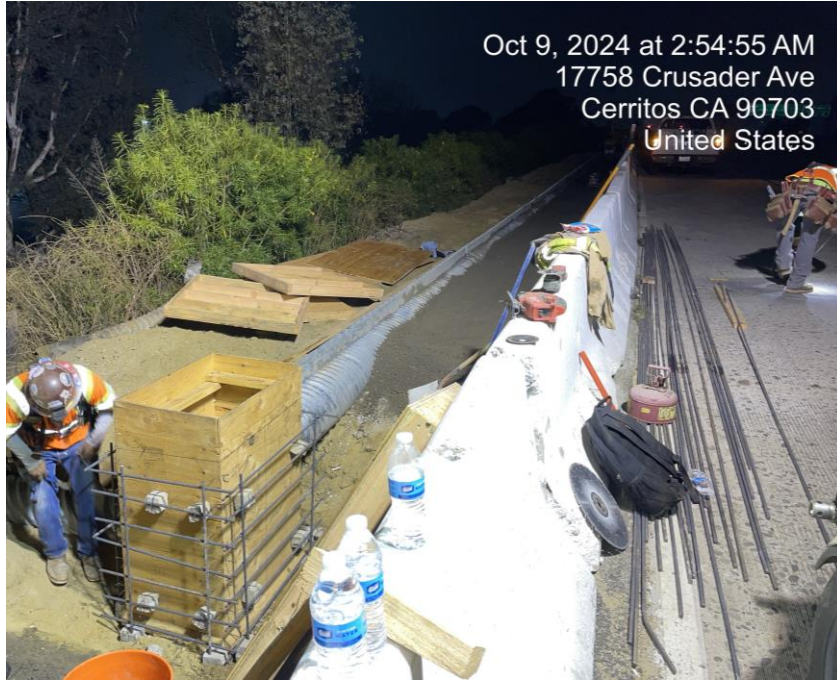
Formation of inlet for connection of pipes of new drainage system
