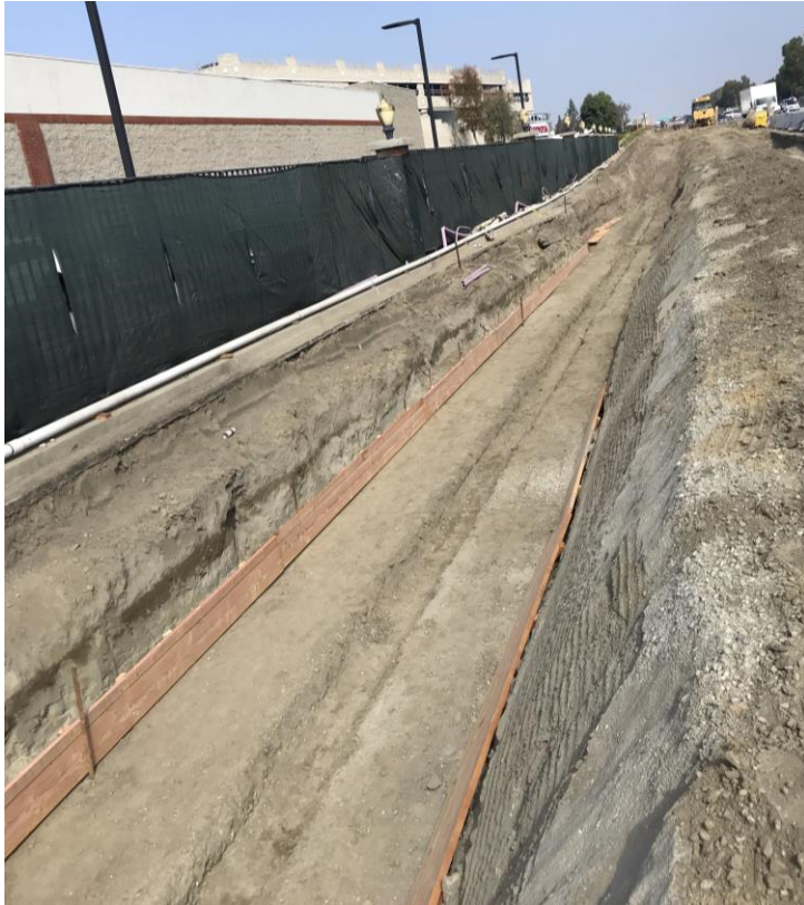
Forming of bottom of retaining wall for the off-ramp
