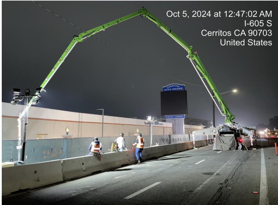
Concrete pour for footing of new retaining wall
