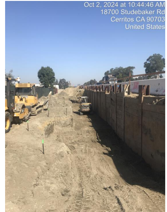
Finalization of shoring of work area
