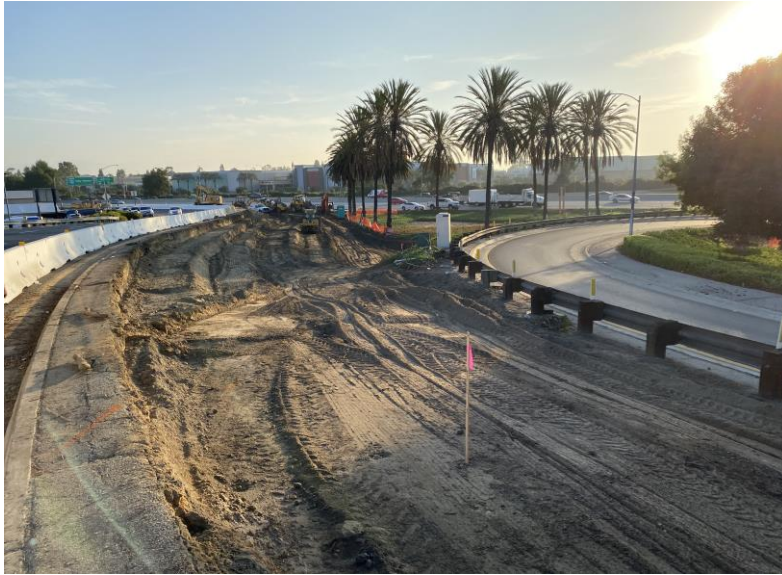
Graded section on left side of off-ramp
