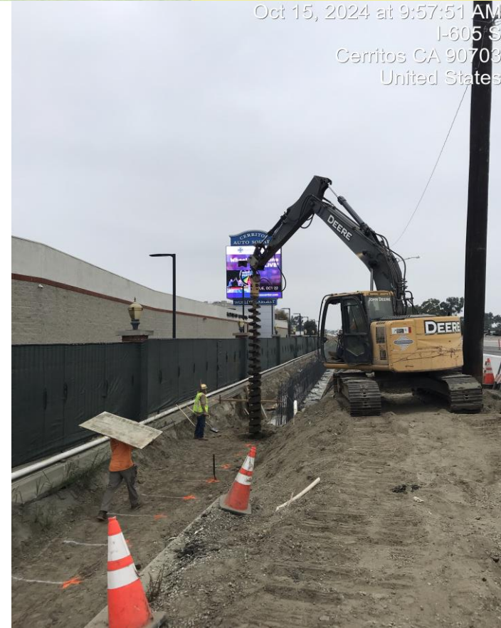
Pile drilling at right of side of South St SB off-ramp
