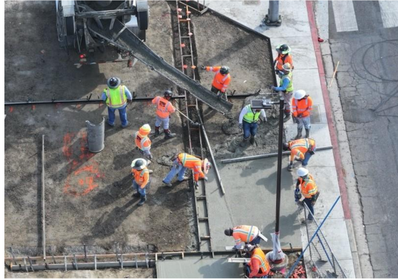
Placing concrete for Mixing Zone construction east overview
