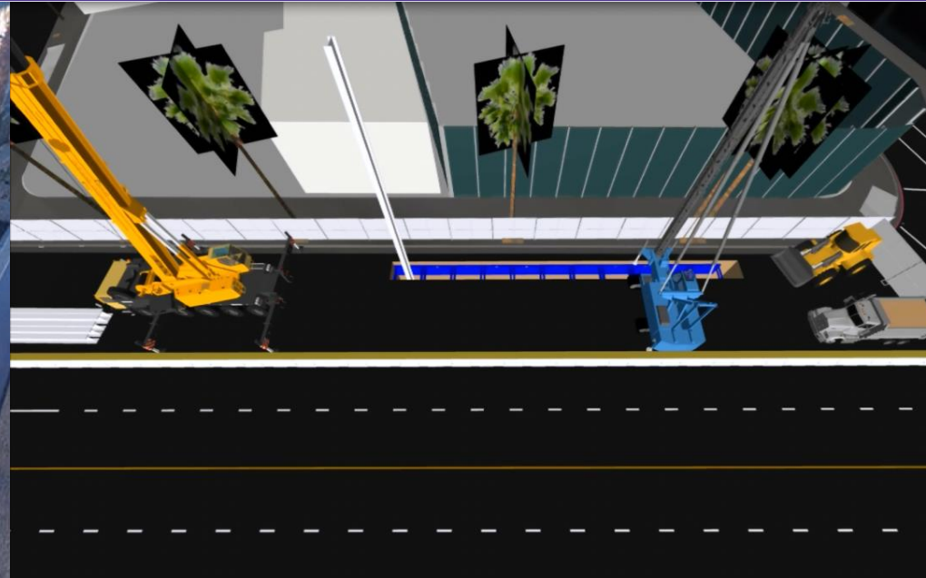
Rendering of work zone showing pile installation
