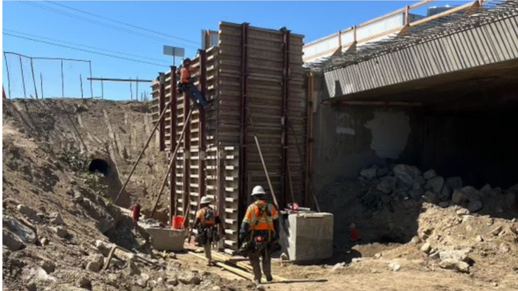
Castaic Creek Bridge, August 2024
