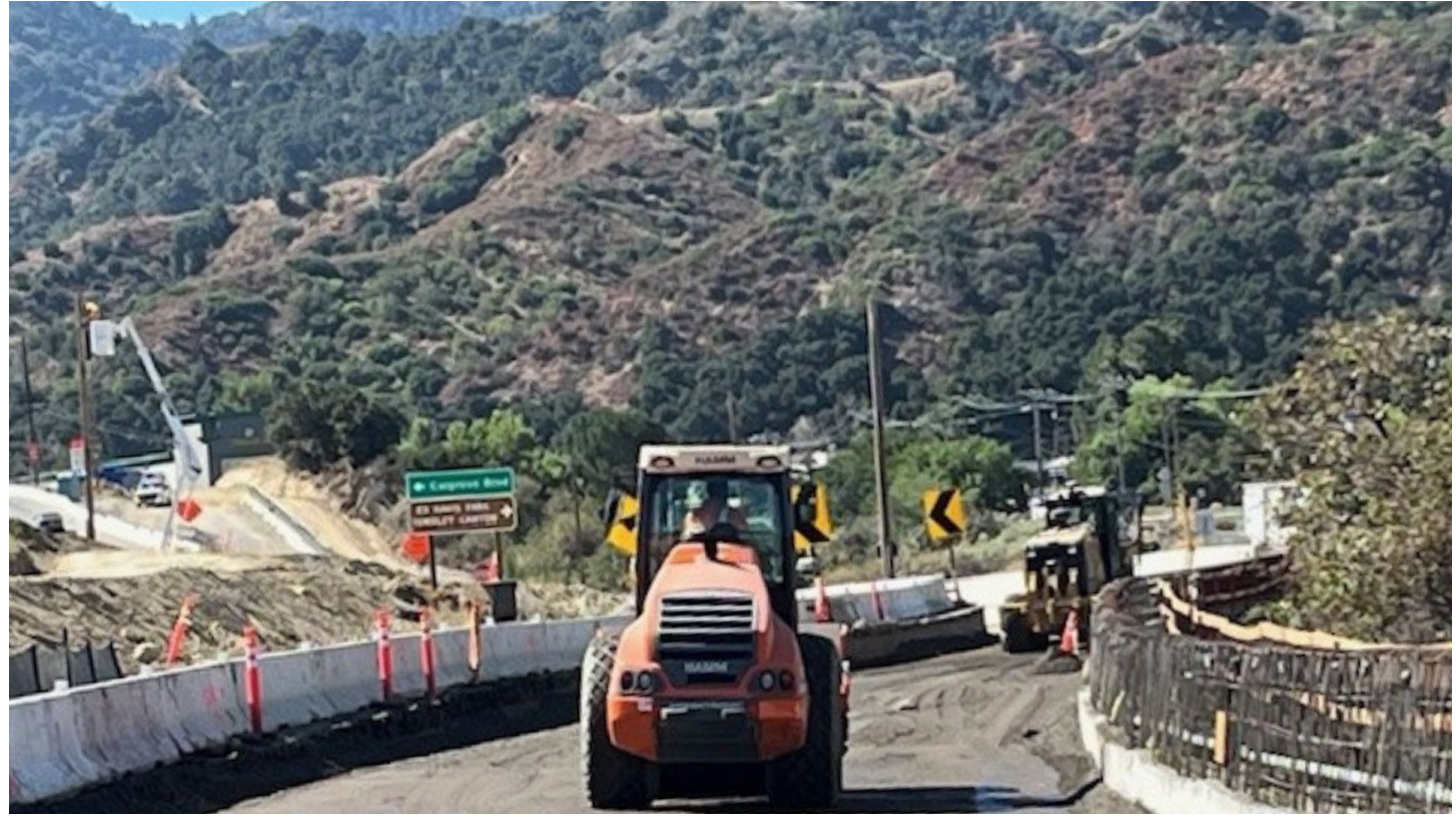
Southbound Calgrove Bl off-ramp
