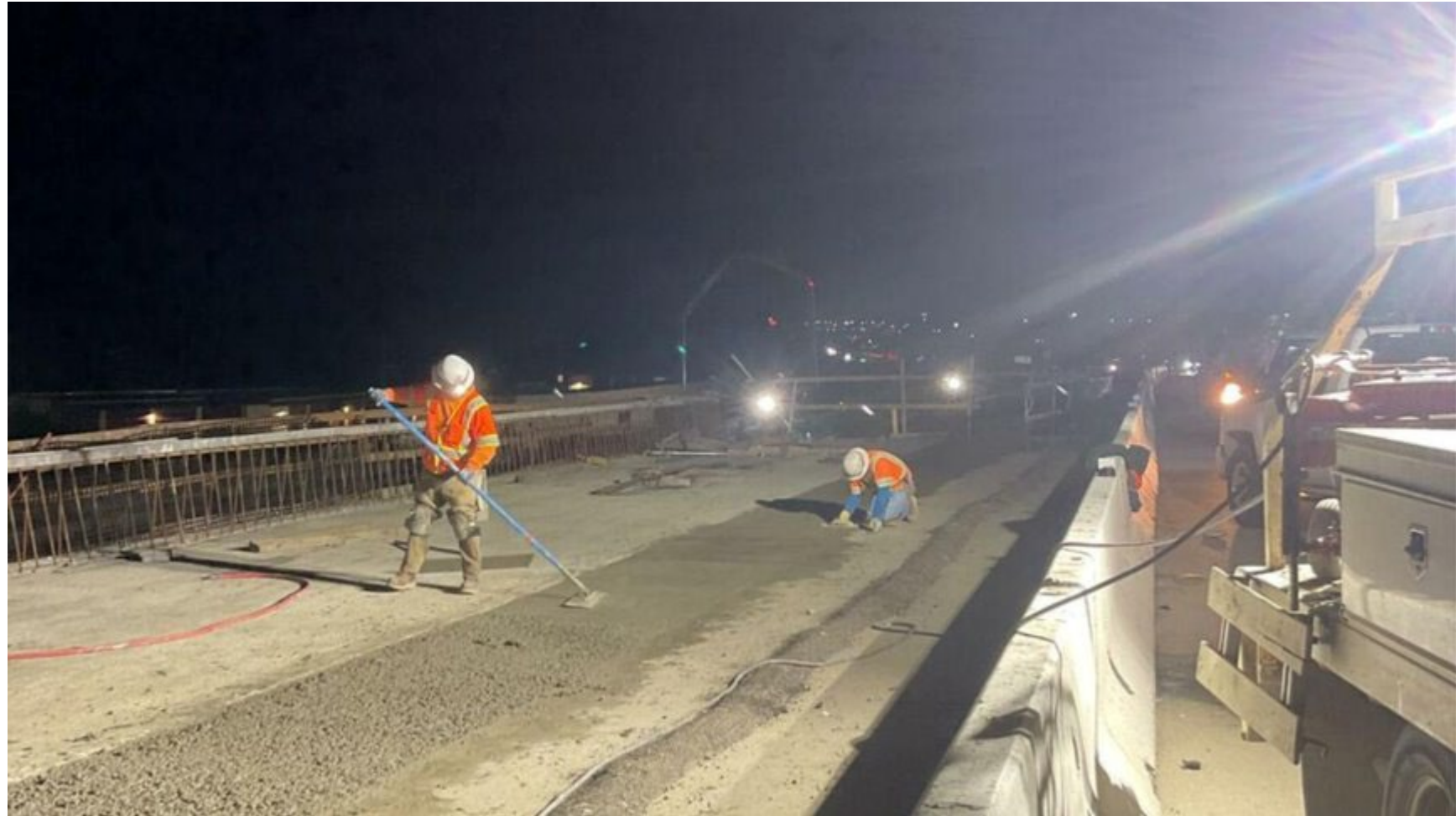
Calgrove BI Bridge concrete setting, June 2024
