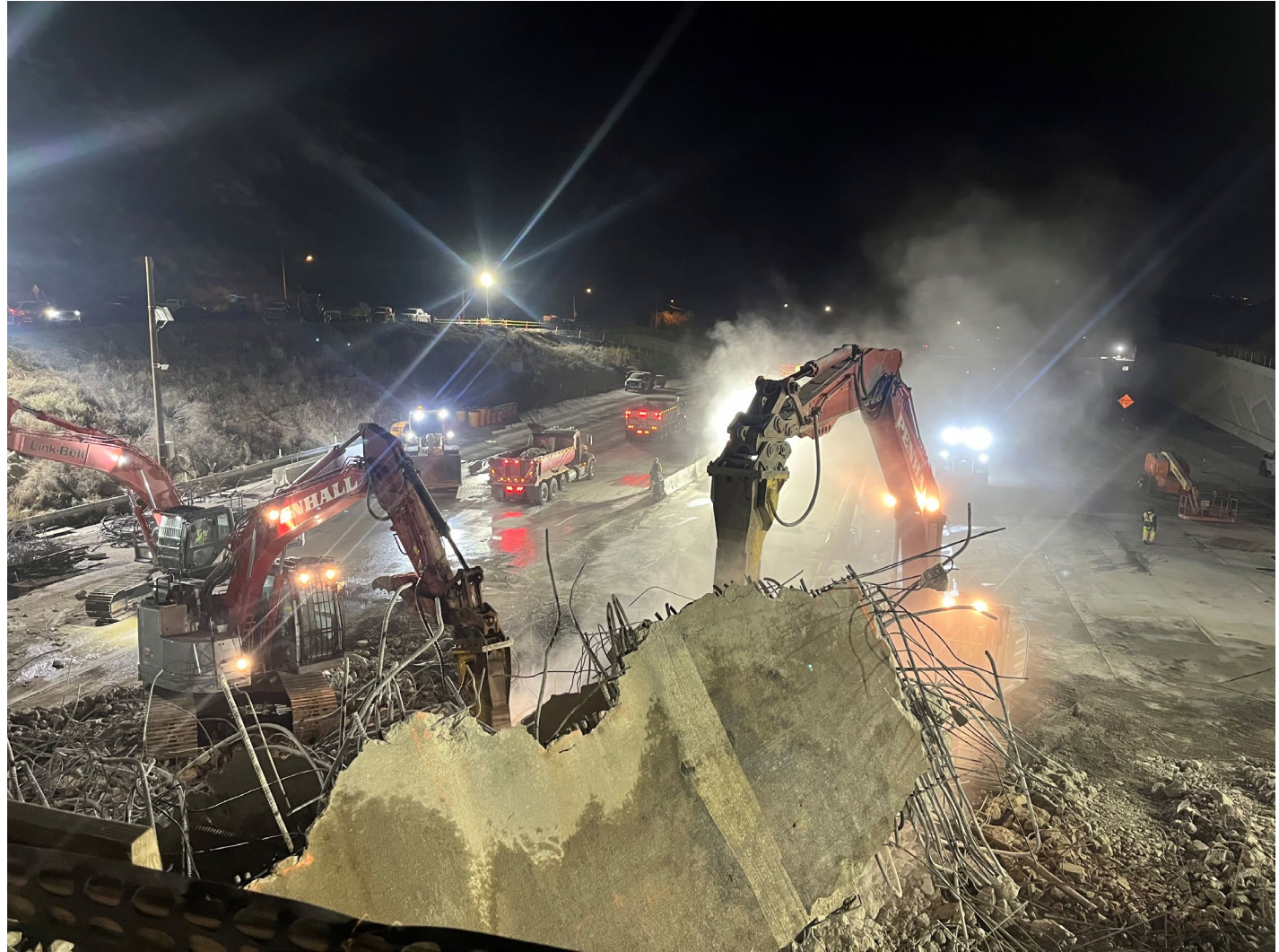
Weldon Canyon Rd Bridge Demolition, November 2023
