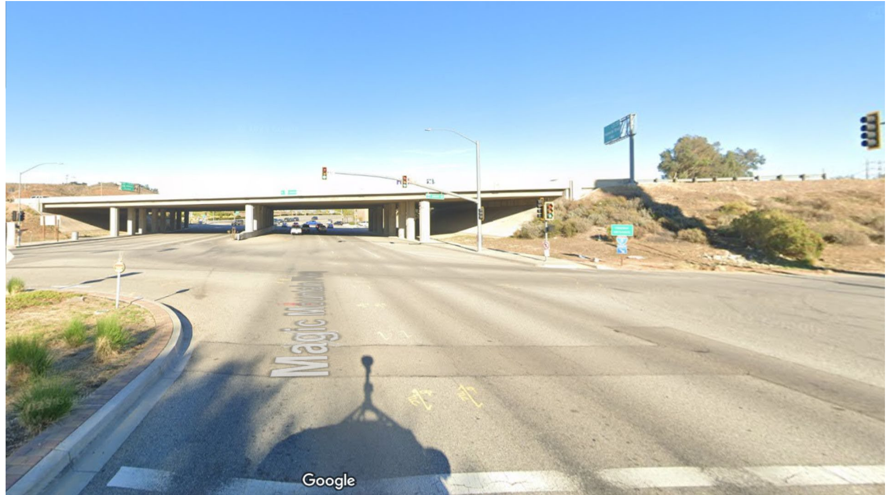
Google Maps image capture of Magic Mountain Pkwy bridge
