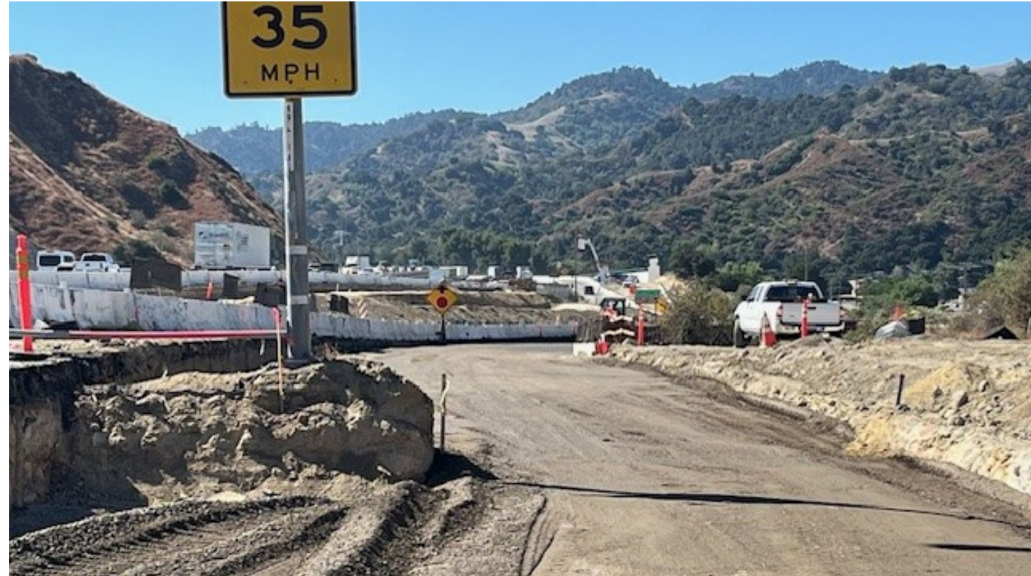
Southbound Calgrove Bl off-ramp
