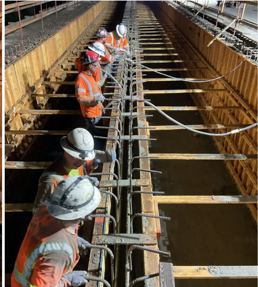
Gavin Canyon Bridge falsework construction and concrete pour, July 2024
