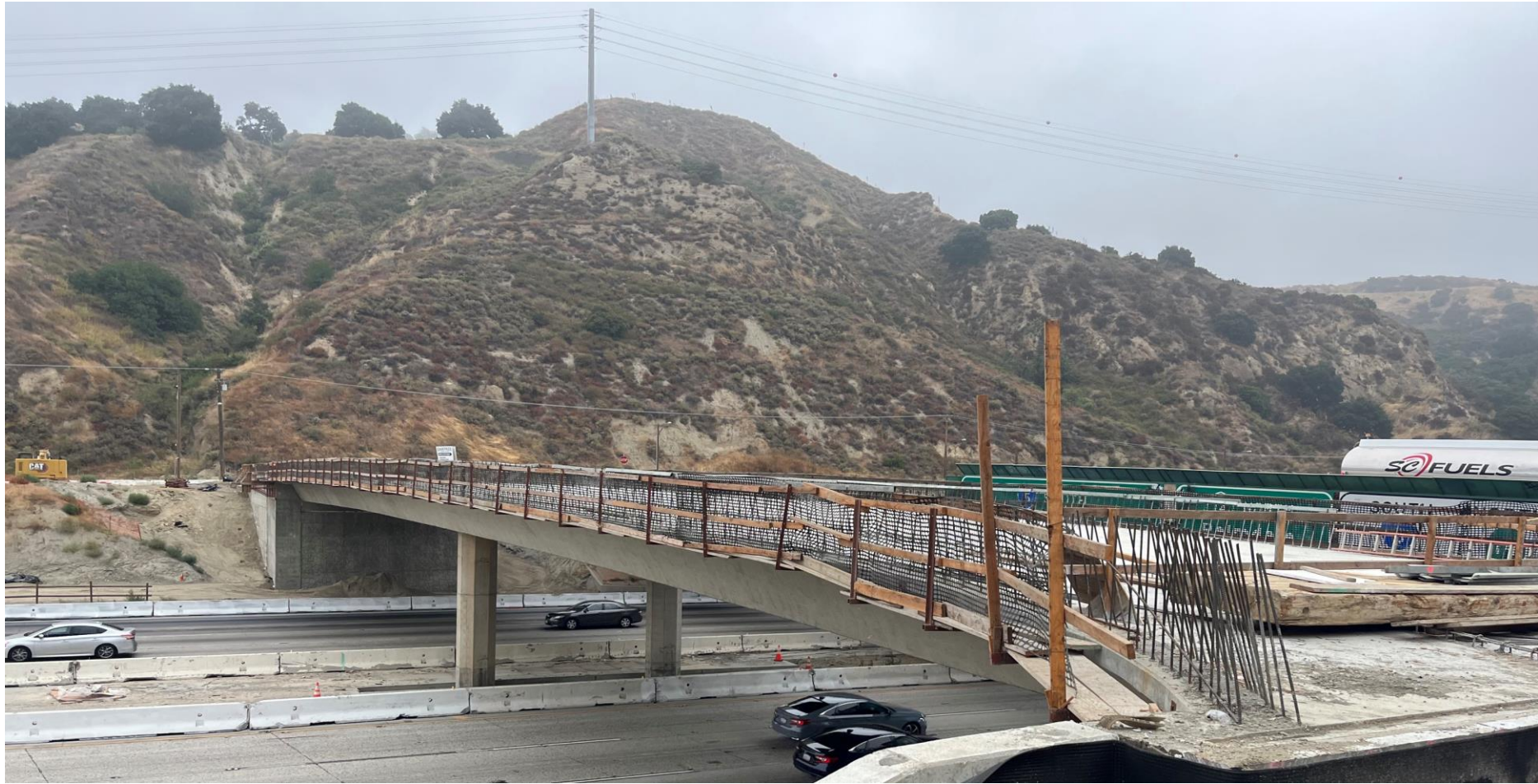
Weldon Canyon Overcrossing bridge construction progress, August 2023
