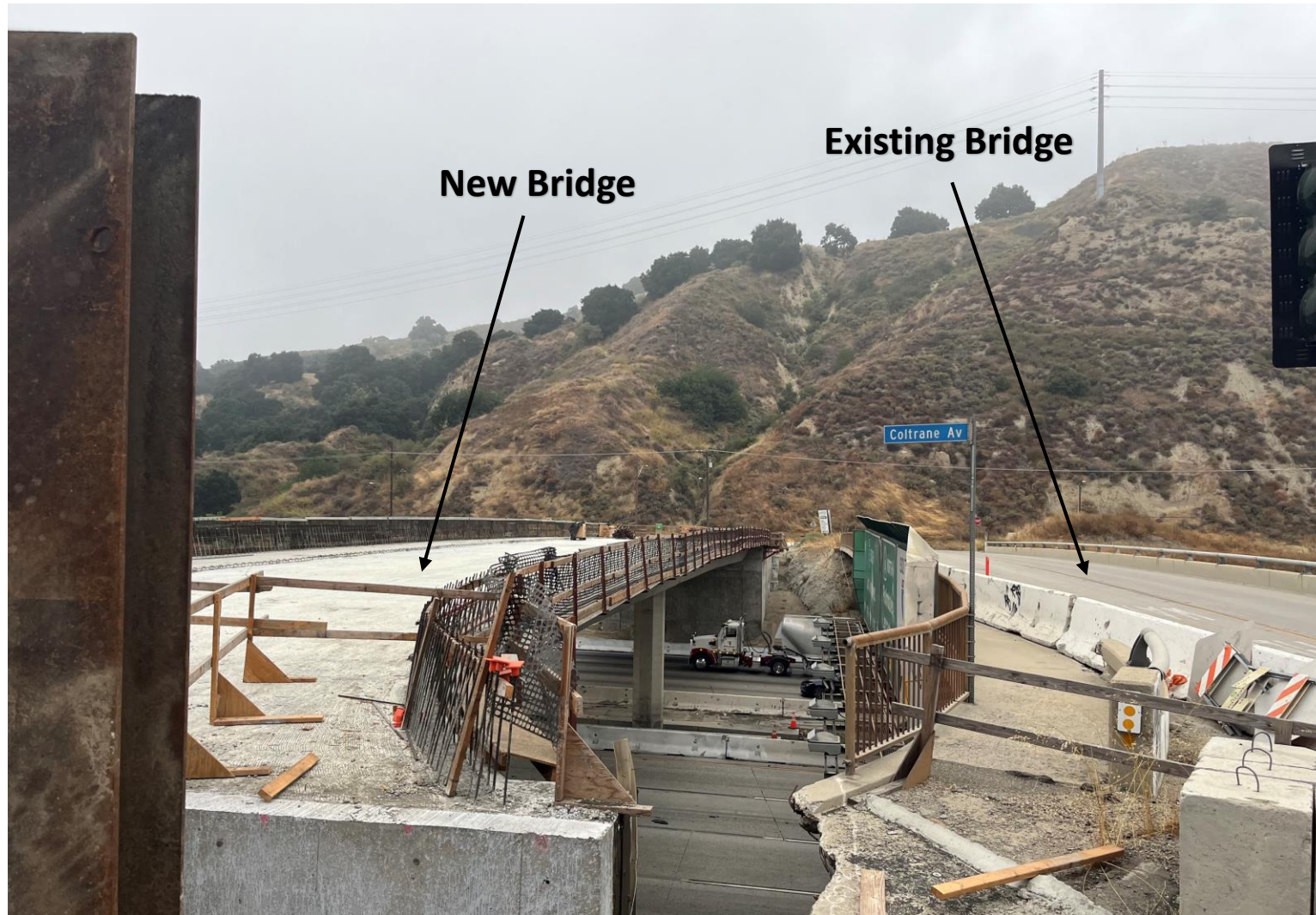
New Weldon Canyon Rd bridge (left), existing Weldon bridge (right), August 2023
