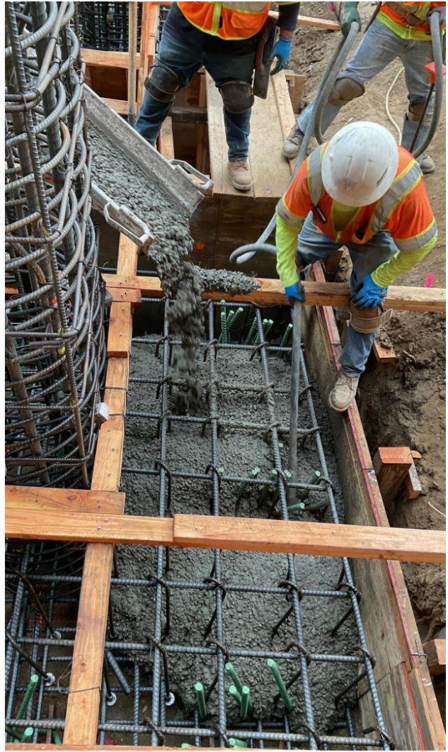
Rebar installation and forming of wingwalls for the new Weldon Canyon Rd Bridge, June 2023
