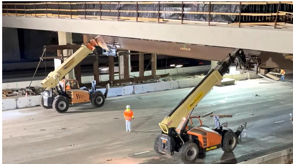
Weldon Canyon Overcrossing bridge falsework removal, May 2023
