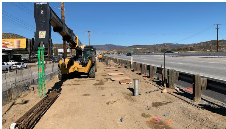
Sound wall construction location (left) and construction activity (right), including drilling, concrete, and rebar work.
