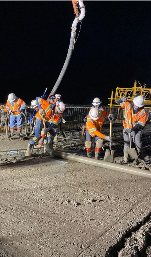
Concrete placement for the new deck on Weldon Canyon Rd bridge in May 2023
