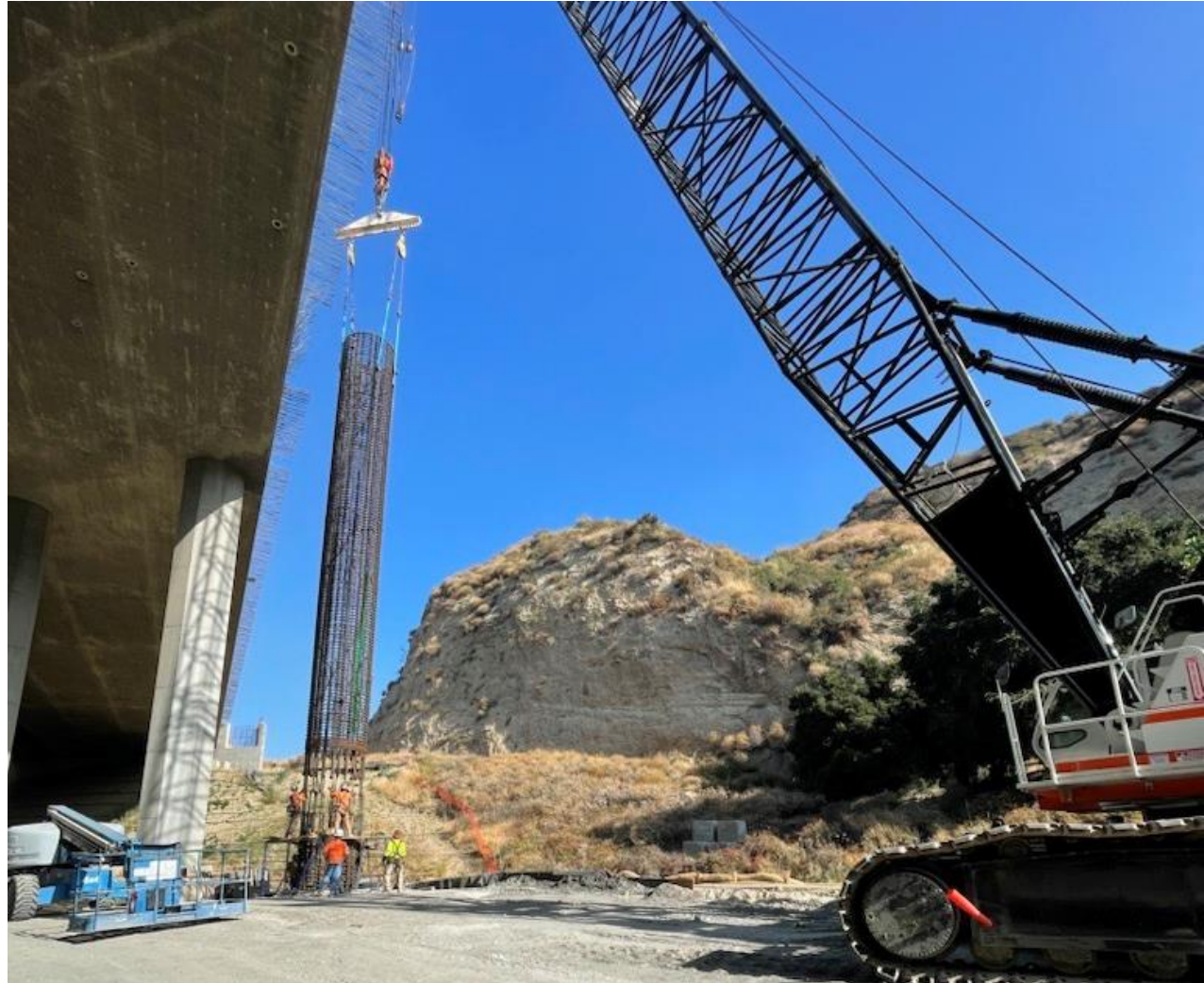
Falsework grading at Gavin Canyon Undercrossing Bridge, August 2023
