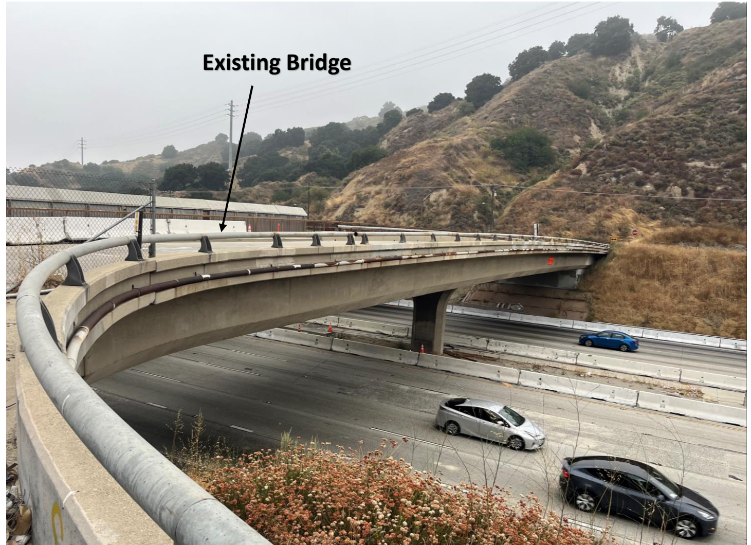
Existing Weldon Canyon Rd Bridge to be demolished
