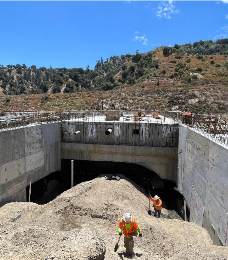
Backfilling of abutments at Weldon Canyon Rd Bridge, August 2023
