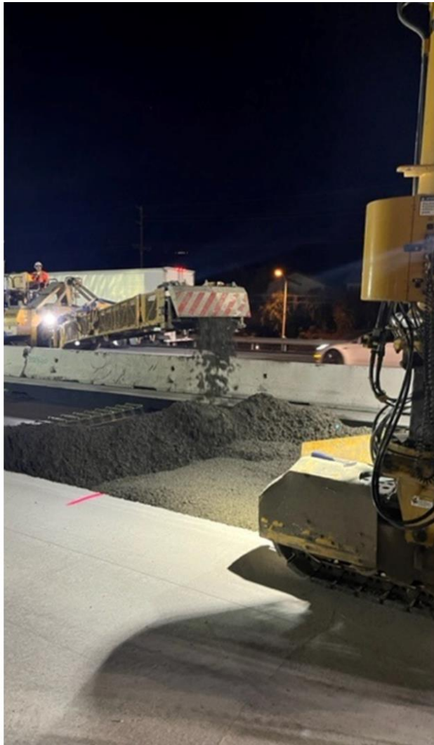
Concrete placement progress in the center median
