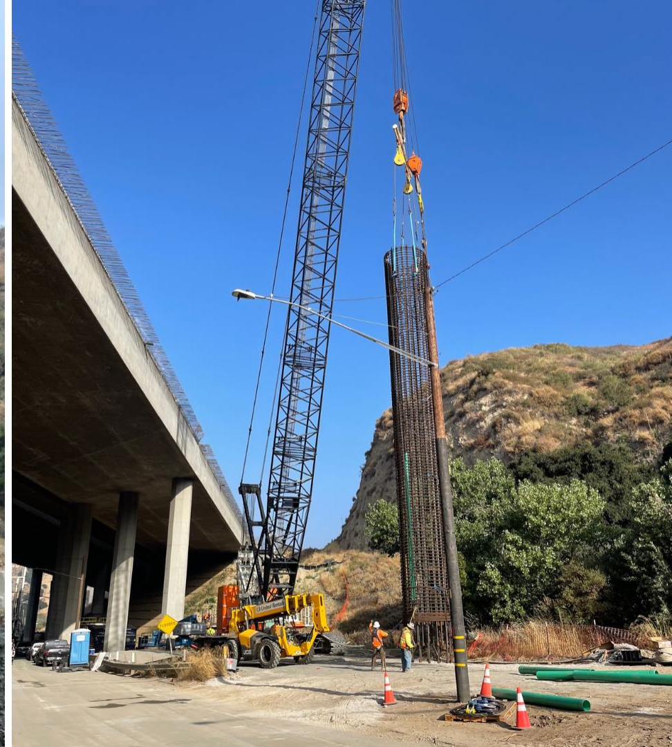
Installation of CIDH cage for Column at Gavin Bridge, August 2023
