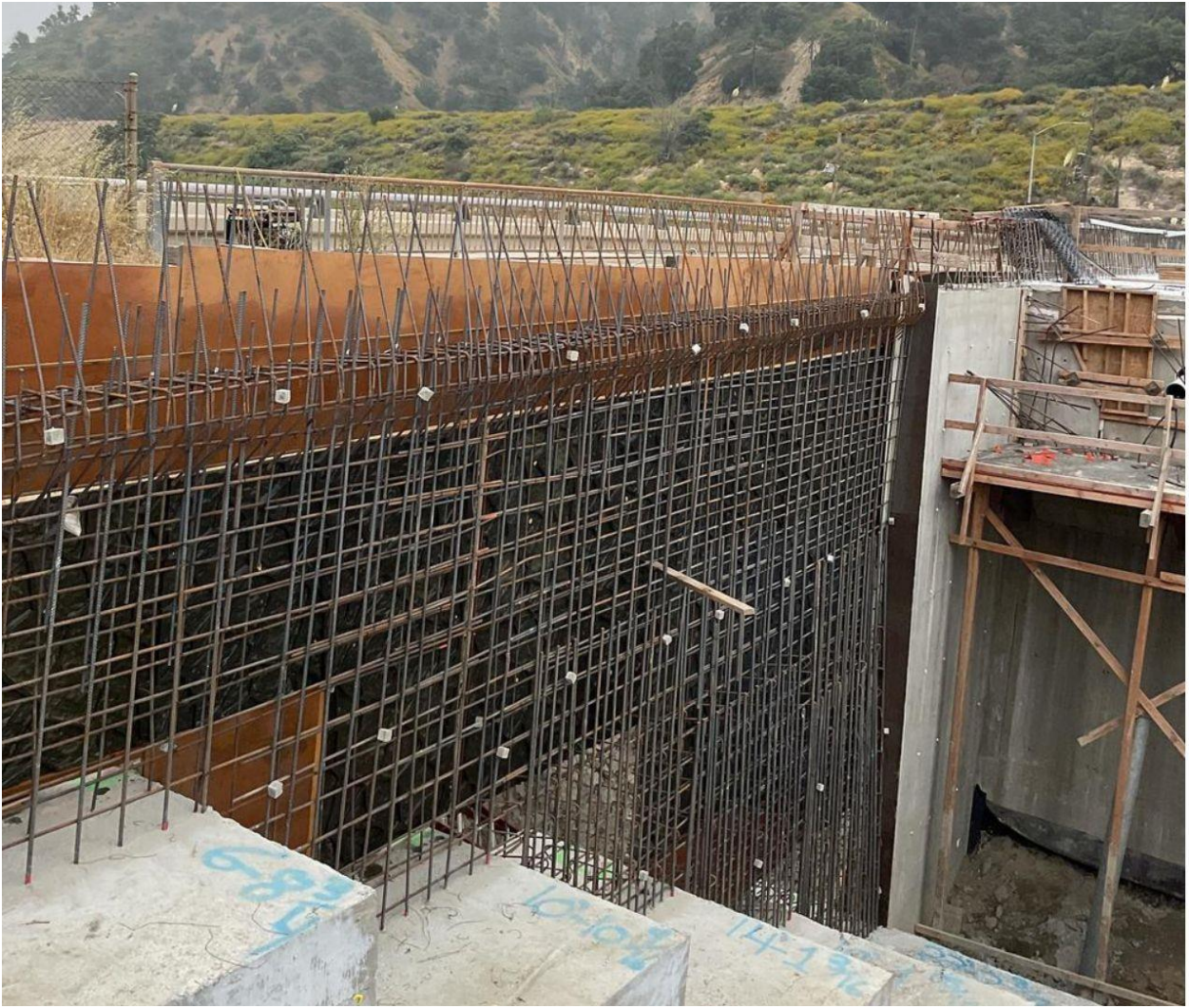
Rebar installation and forming of wingwalls for the new Weldon Canyon Rd Bridge, June 2023
