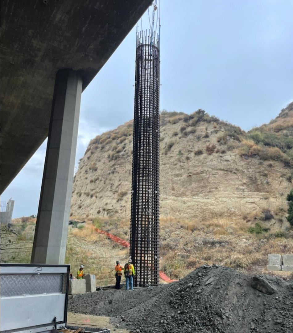
Installation of CIDH cage for Column at Gavin Bridge, August 2023
