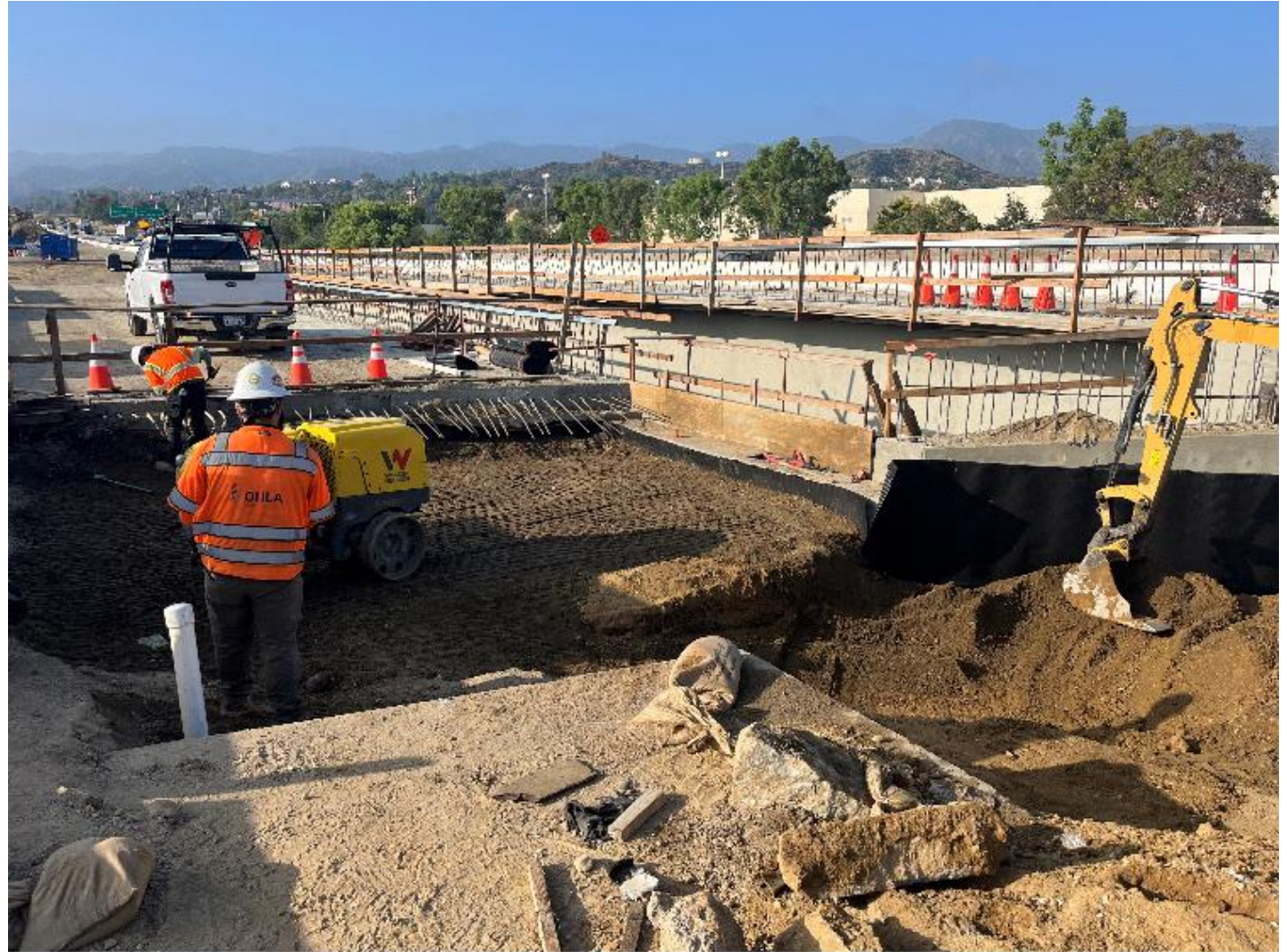
Progress photo of Abutment at Butte Canyon Bridge, August 2023
