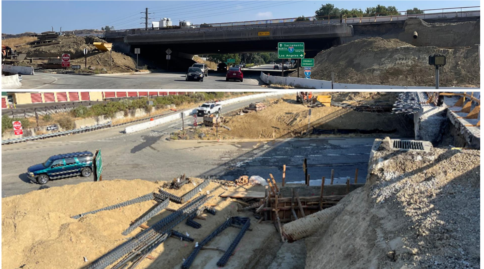
Calgrove BI Undercrossing bridge progress, August 2023
