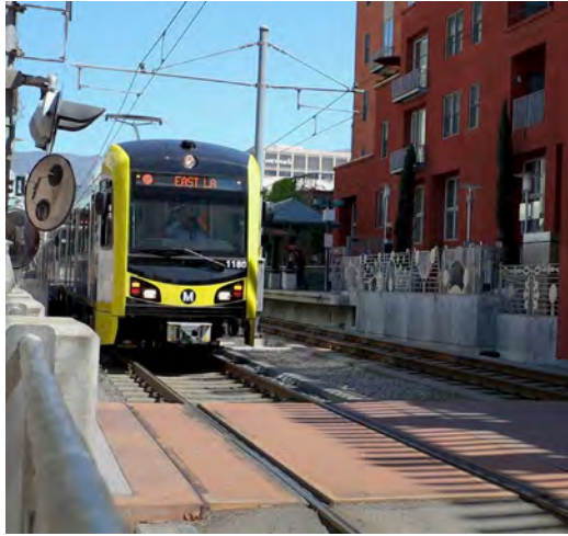
Overhead Catenary System Poles
