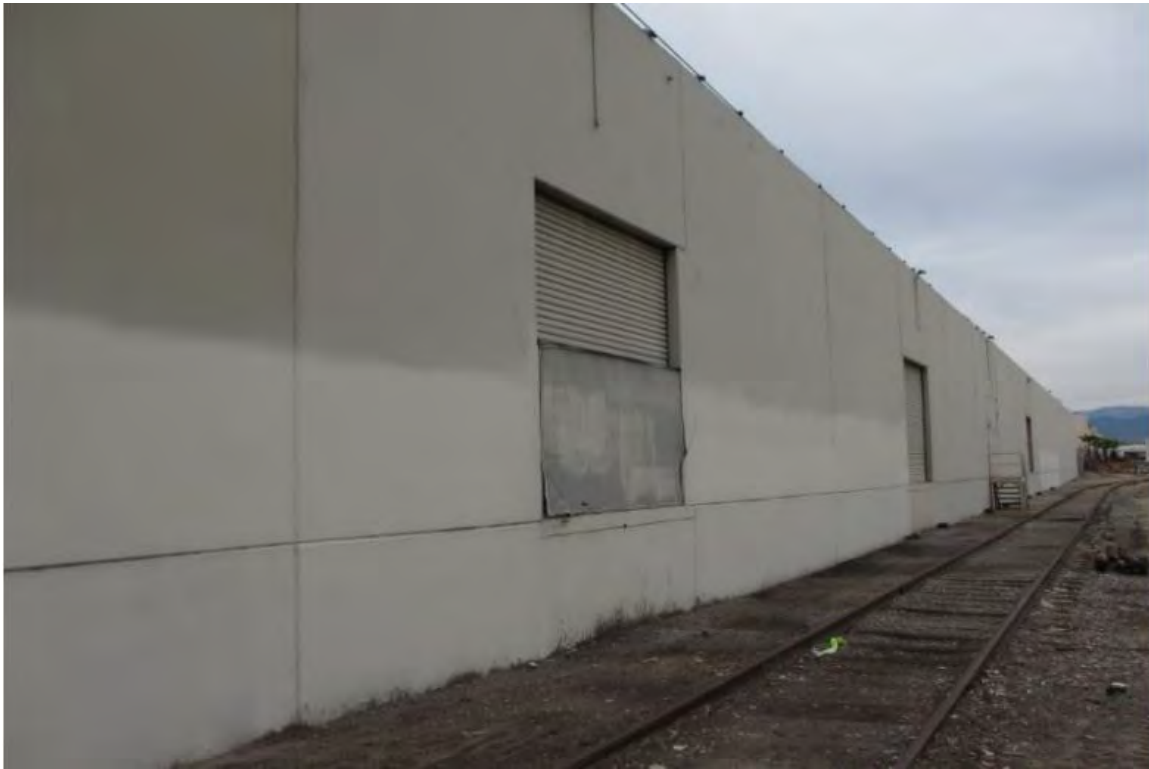
Figure 3.4.6. Goodyear Tire and Rubber Company Warehouse Constructed 1952 and Existing Rail Alignment Facing Washington Boulevard (2353 Garfield Avenue) (View east). Existing Rail Alignment North of Goodyear Tire and Rubber Company Warehouse at Washington Boulevard (View north)
