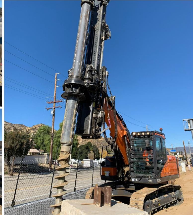
Sound wall construction location (left) and construction activity (right), including drilling, concrete, and rebar work.
