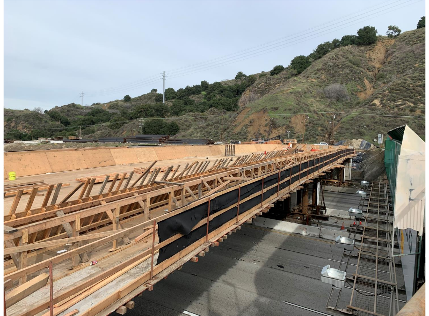
Weldon Canyon Rd Bridge falsework installation (temporary structures)
