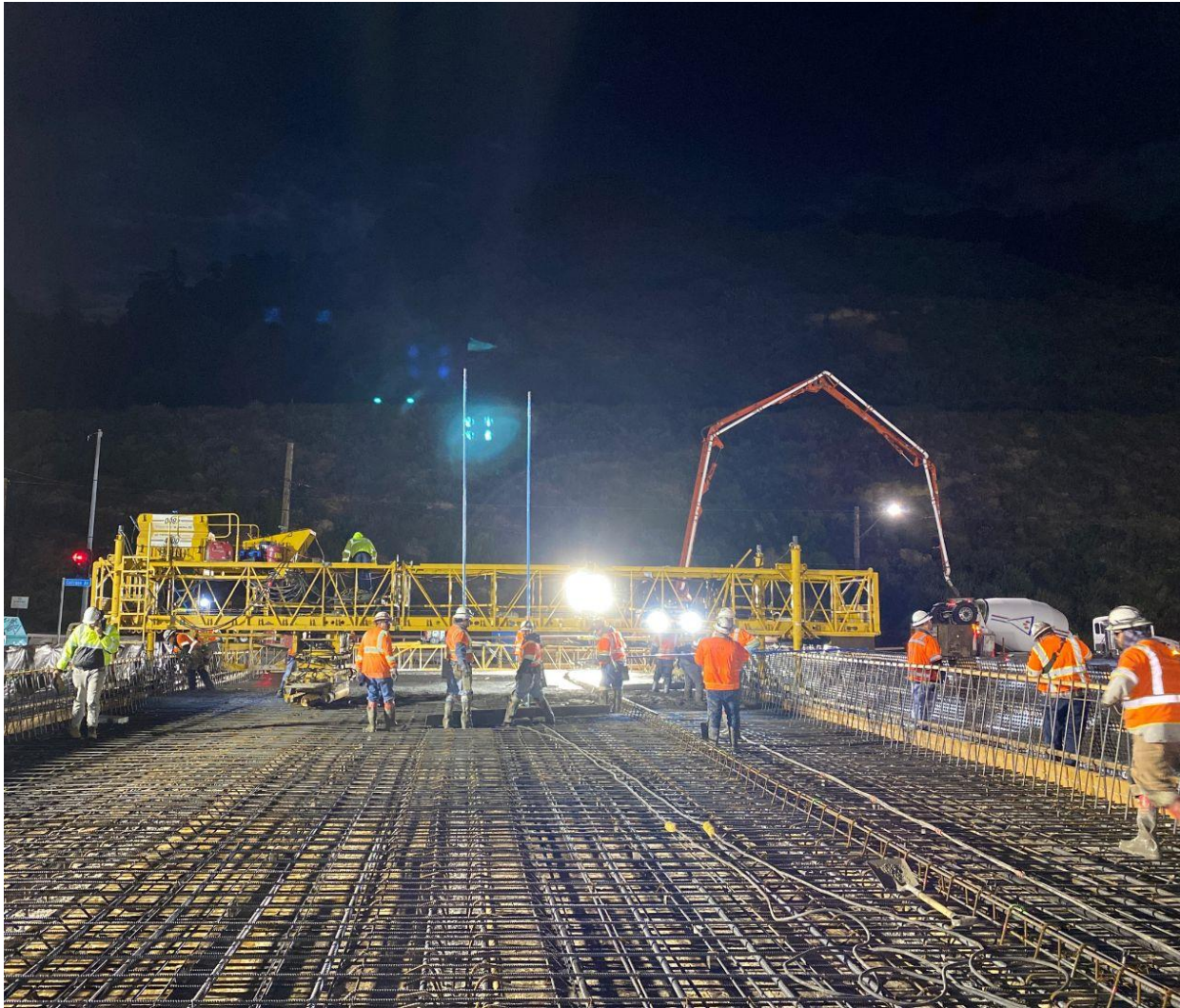
Concrete placement for the new deck on Weldon Canyon Rd bridge in May 2023
