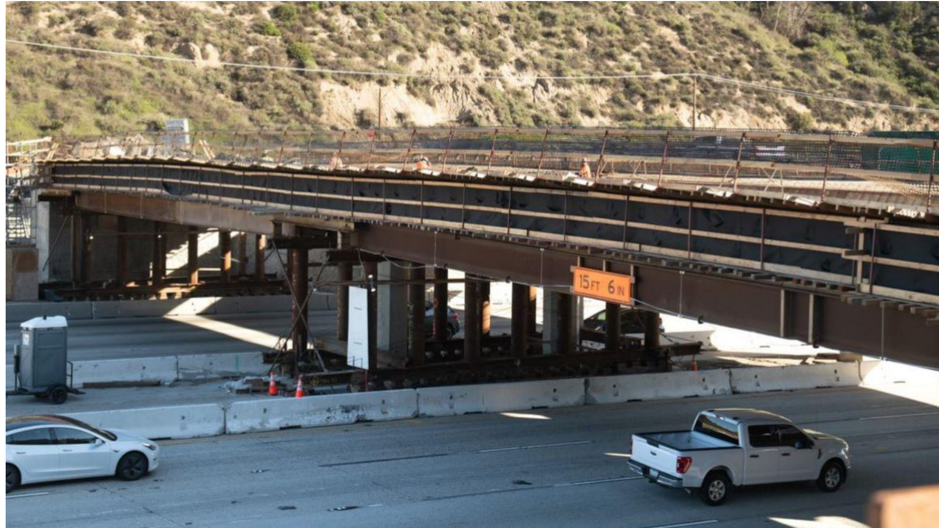
Weldon Canyon Overcrossing bridge construction progress through April 2023
