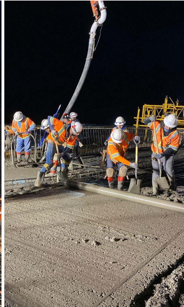
Concrete placement for the new deck on Weldon Canyon Rd bridge in May 2023
