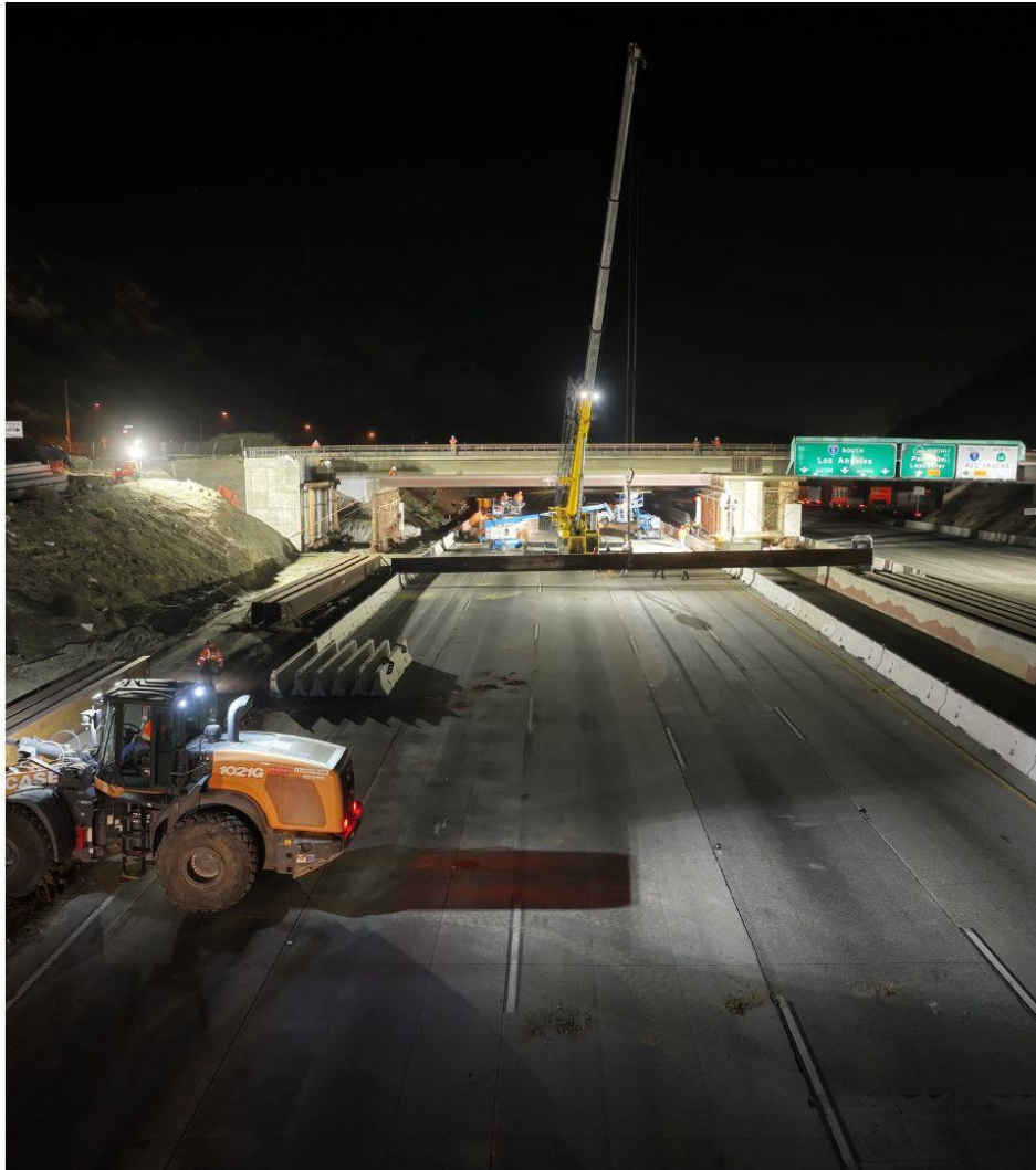
Weldon Canyon Overcrossing bridge falsework installation, November 2022
