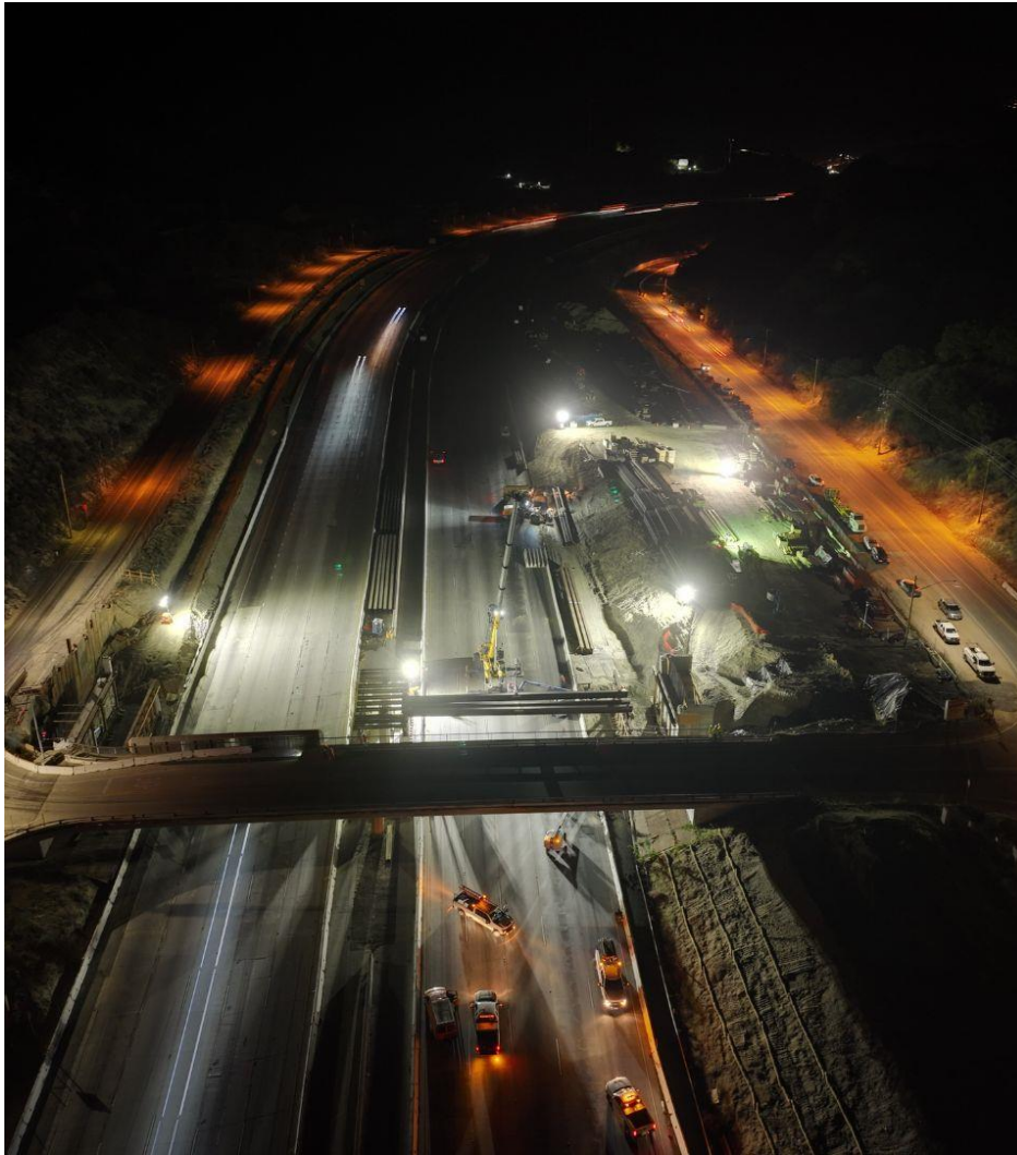
Weldon Canyon Overcrossing bridge falsework installation, November 2022
