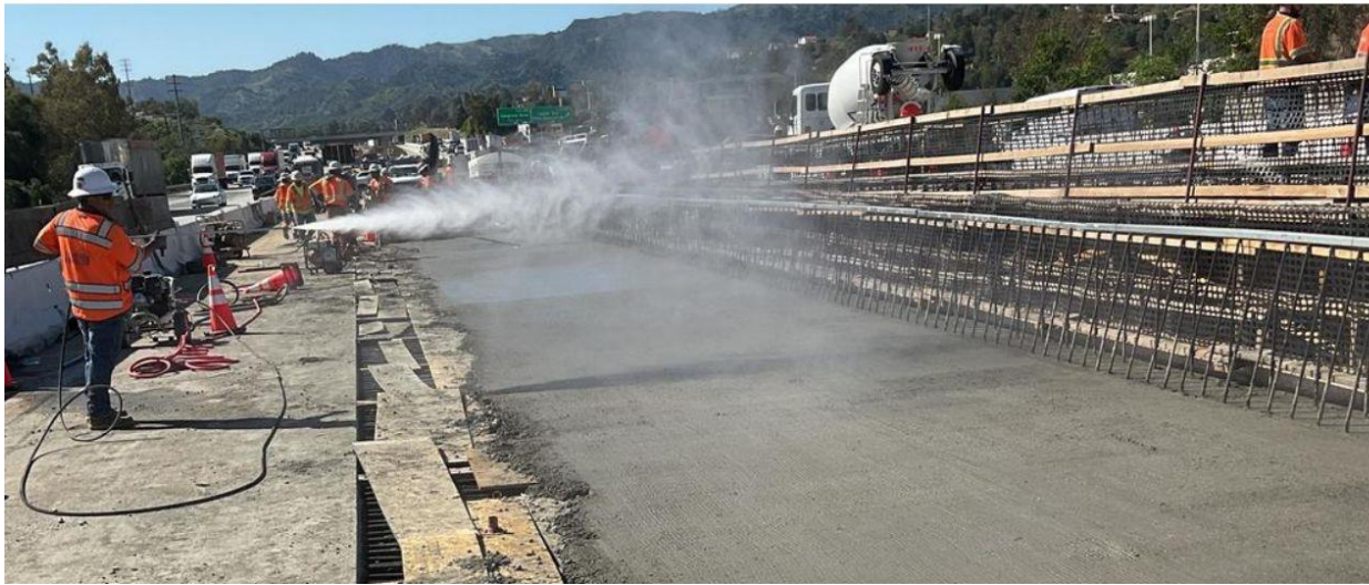
Center median construction activities including excavation, backfill, rebar and concrete work.
