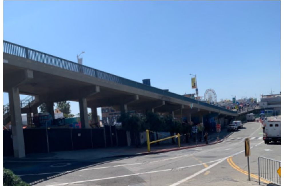
Santa Monica Pier Bridge 53C1900
