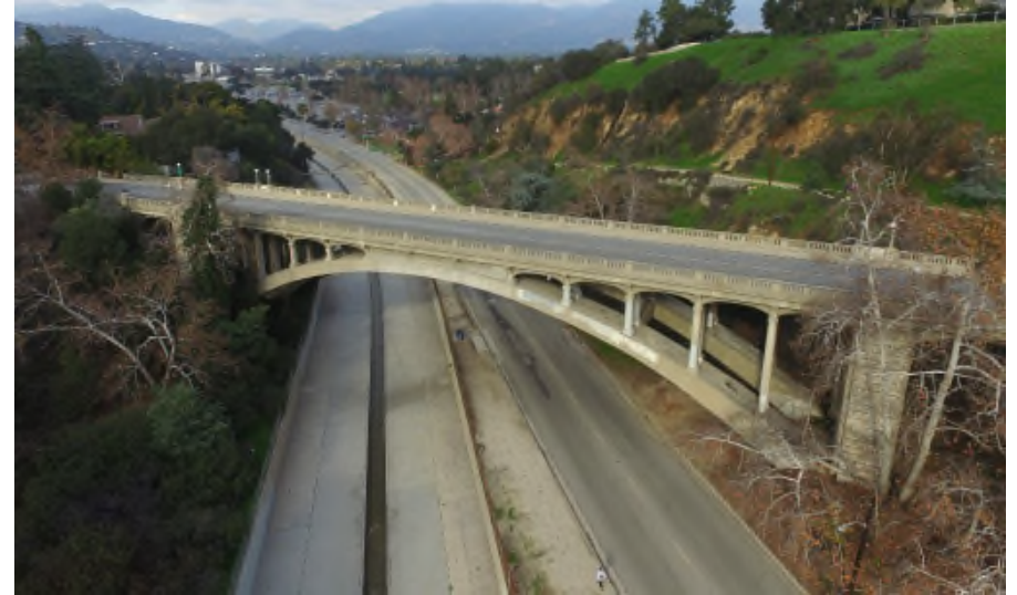
Holly Street Bridge 53C1041
