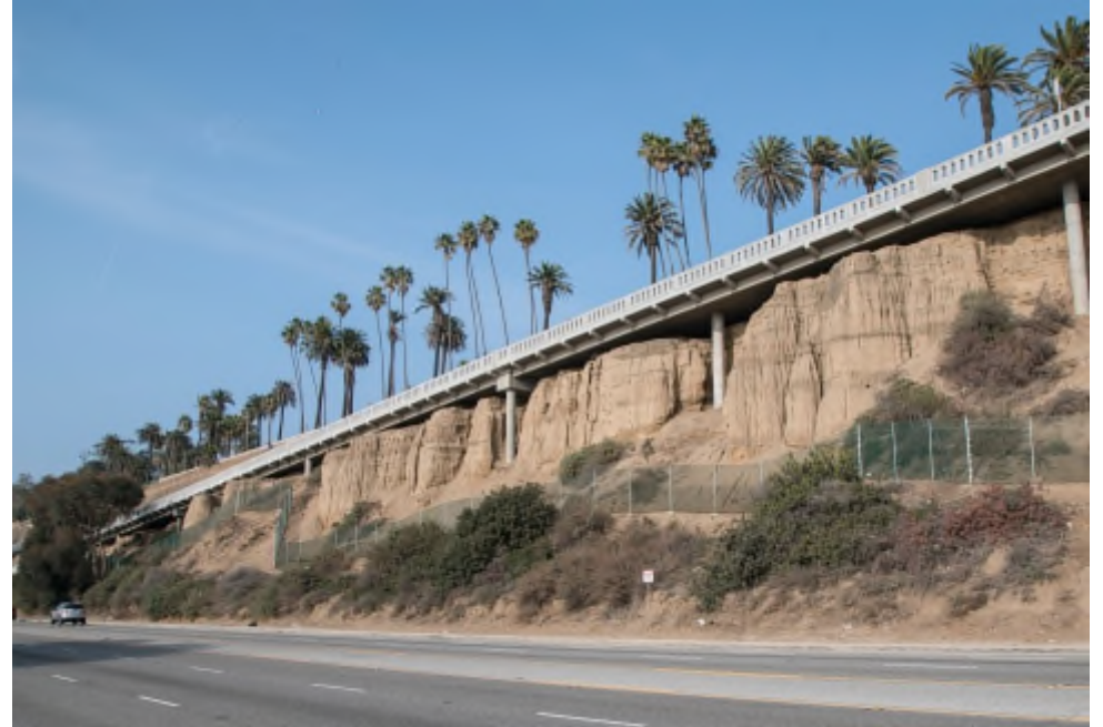
CA Incline Bridge 53C0543
