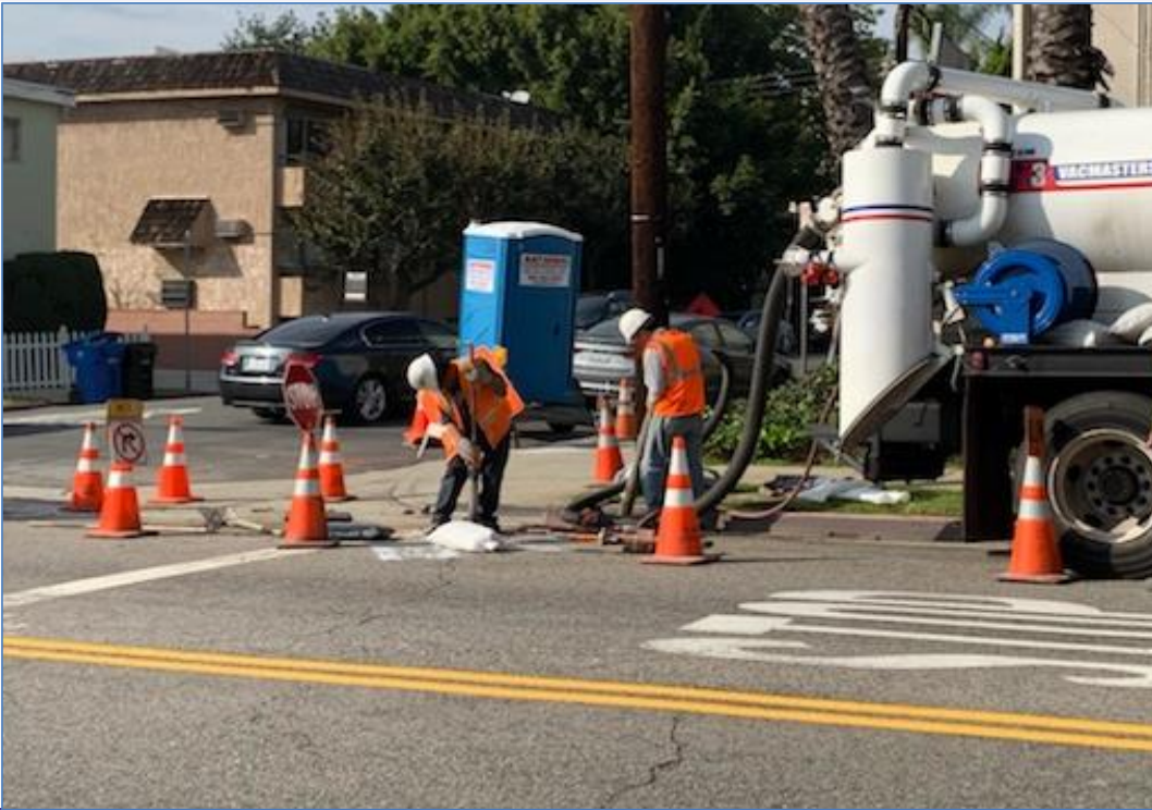
Potholing near Ohio & Federal is complete
