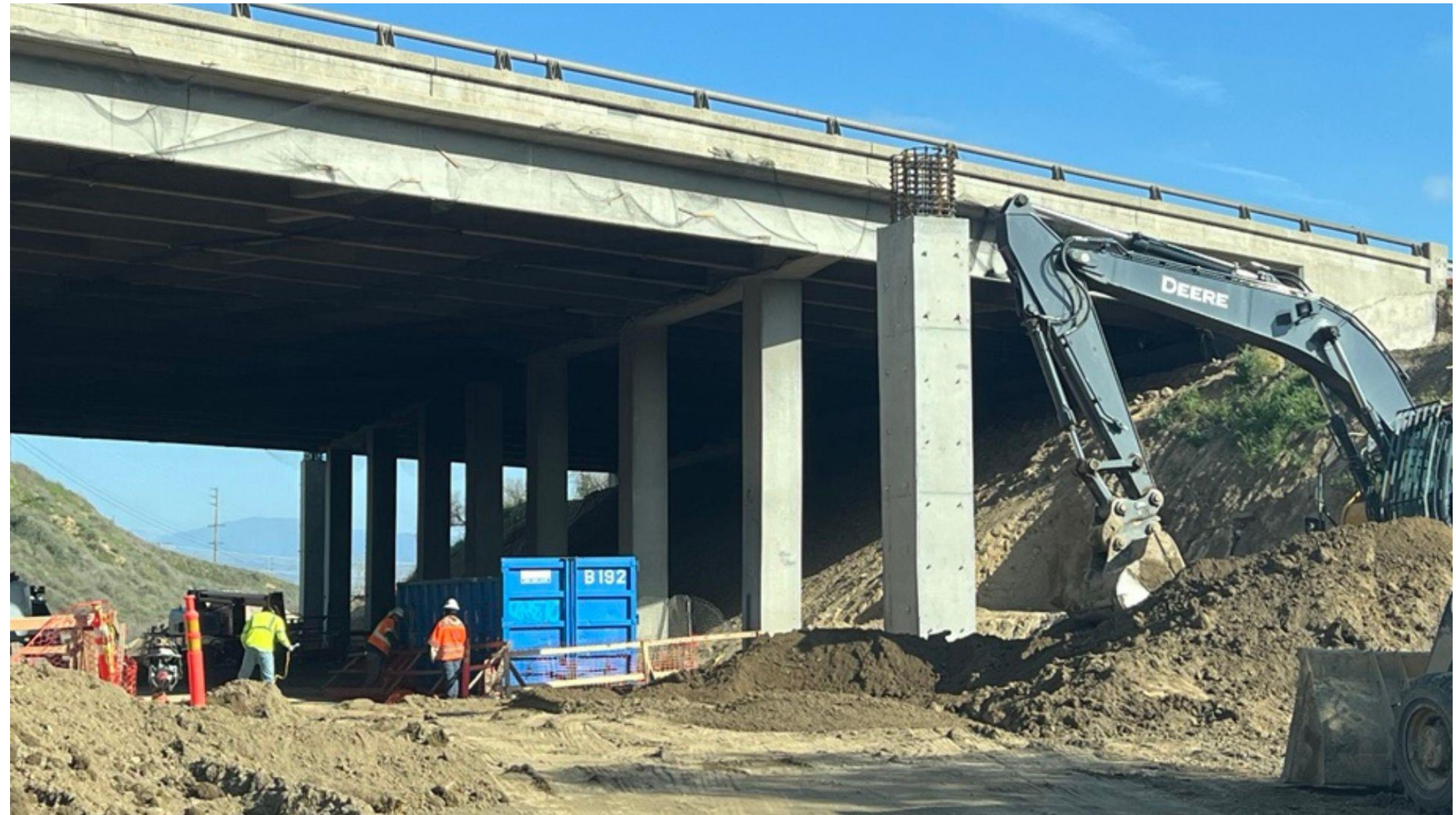
Santa Clara River Overhead Crossing bike path, February 2024
