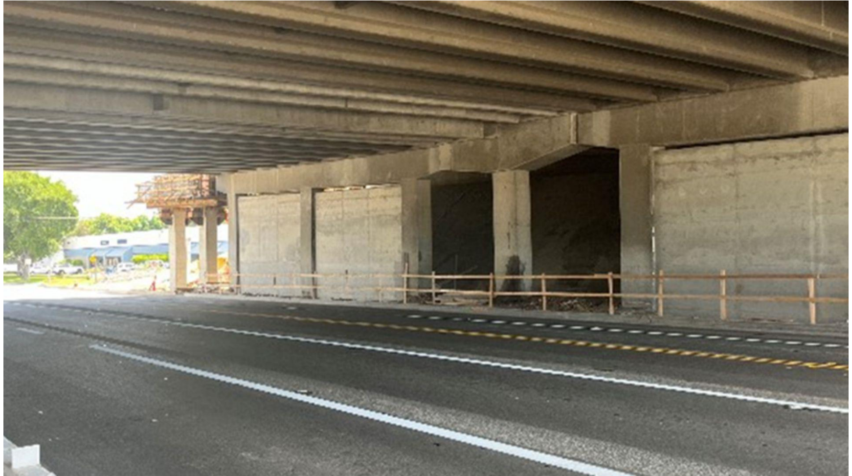
Rye Canyon Rd Bridge, January 2024
