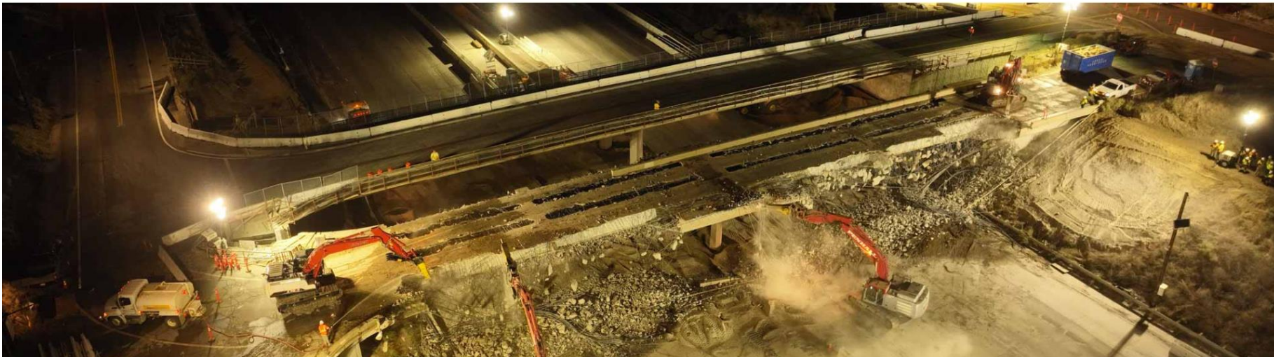
Aerial action photos of Weldon Canyon Overcrossing bridge demolition, November 4, 2023
