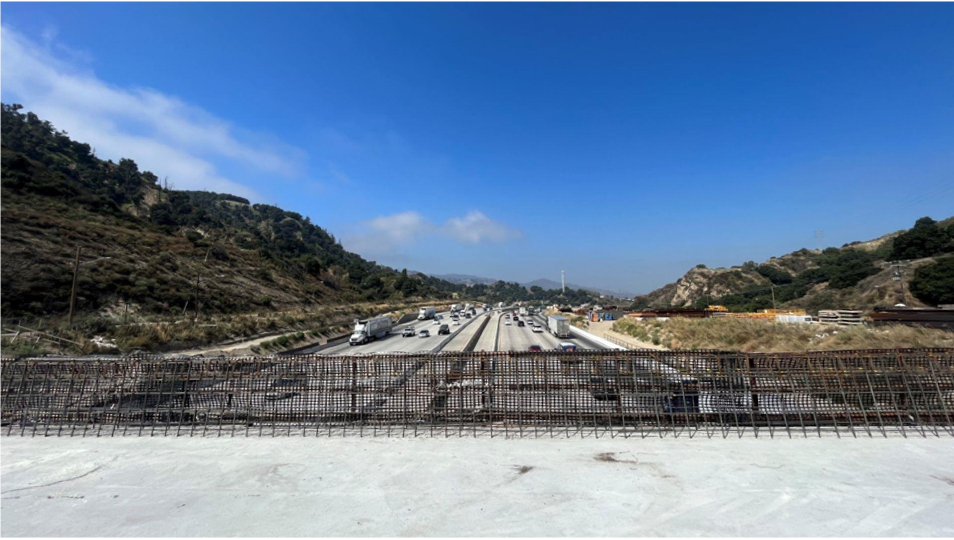
Weldon Canyon Rd bridge barrier installation, November 2023
