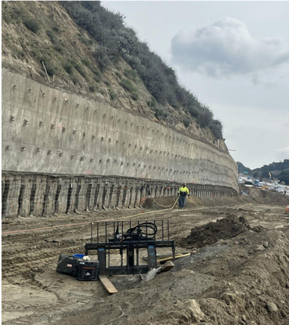
Retaining and soil nail wall construction, January 2024
