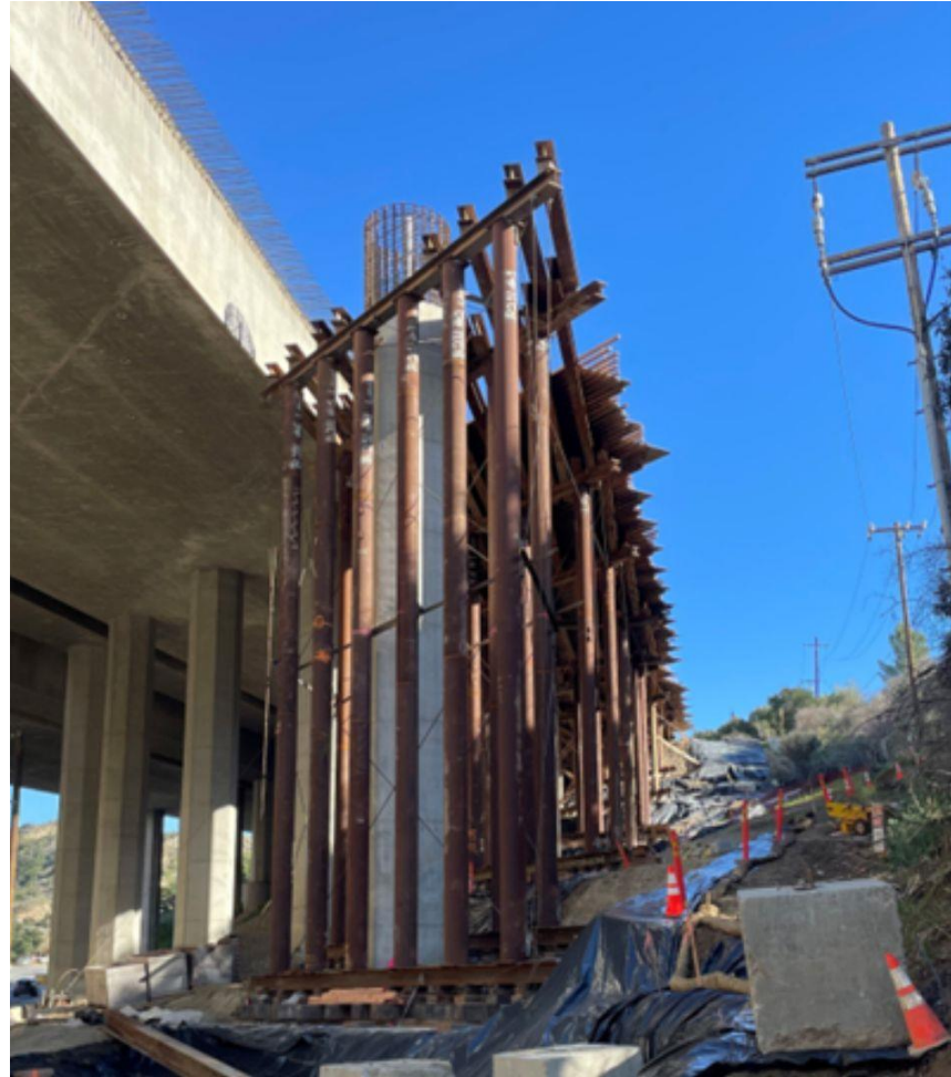
Falsework grading at Gavin Bridge, January 2024
