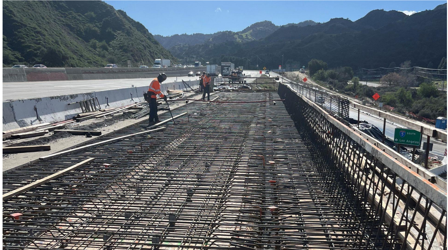
Calgrove BI Undercrossing bridge January 2024
