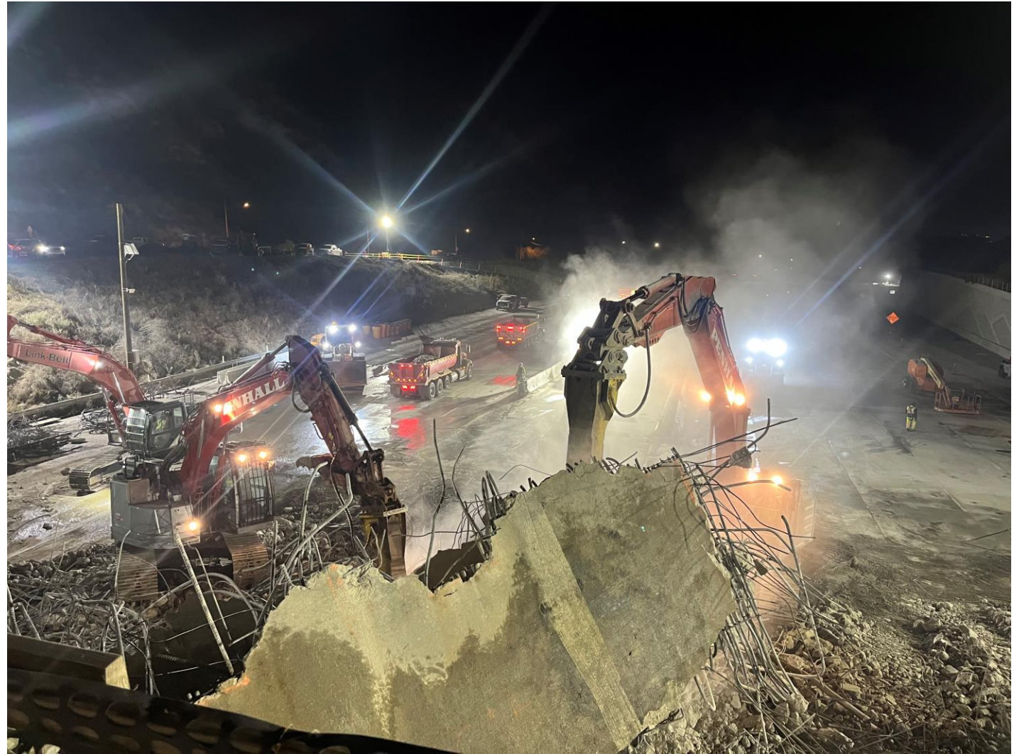
Weldon Canyon Rd Bridge Demolition, November 2023
