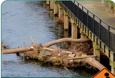
Removing Drift Piling on Bridges
