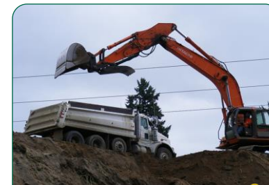
Replacing Embankment Fill
