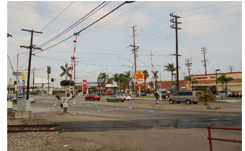
Grade Crossing at Manchester.
