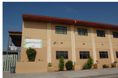
Schools adjacent to the LRT raise the awareness regarding pedestrian safety and measures that must be in place to ensure safe LRT operations and pedestrian paths.
