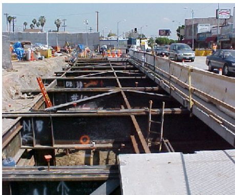
Cut and Cover Construction Goldline Eastside Extension
