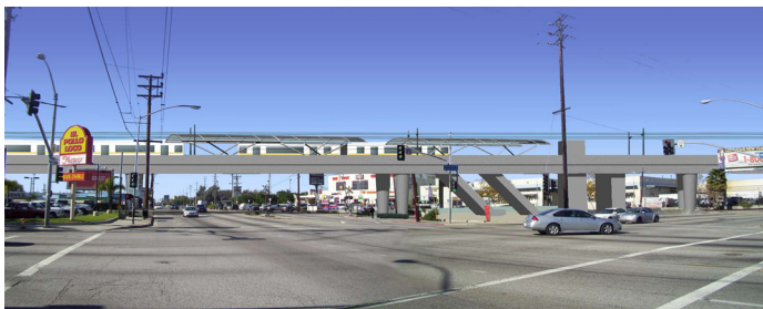
Aerial structure across Manchester Avenue.
