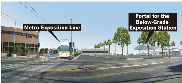
Rendering of portal for the below-grade Crenshaw/Exposition Station that is adjacent to the operation of the at-grade Exposition Line.
