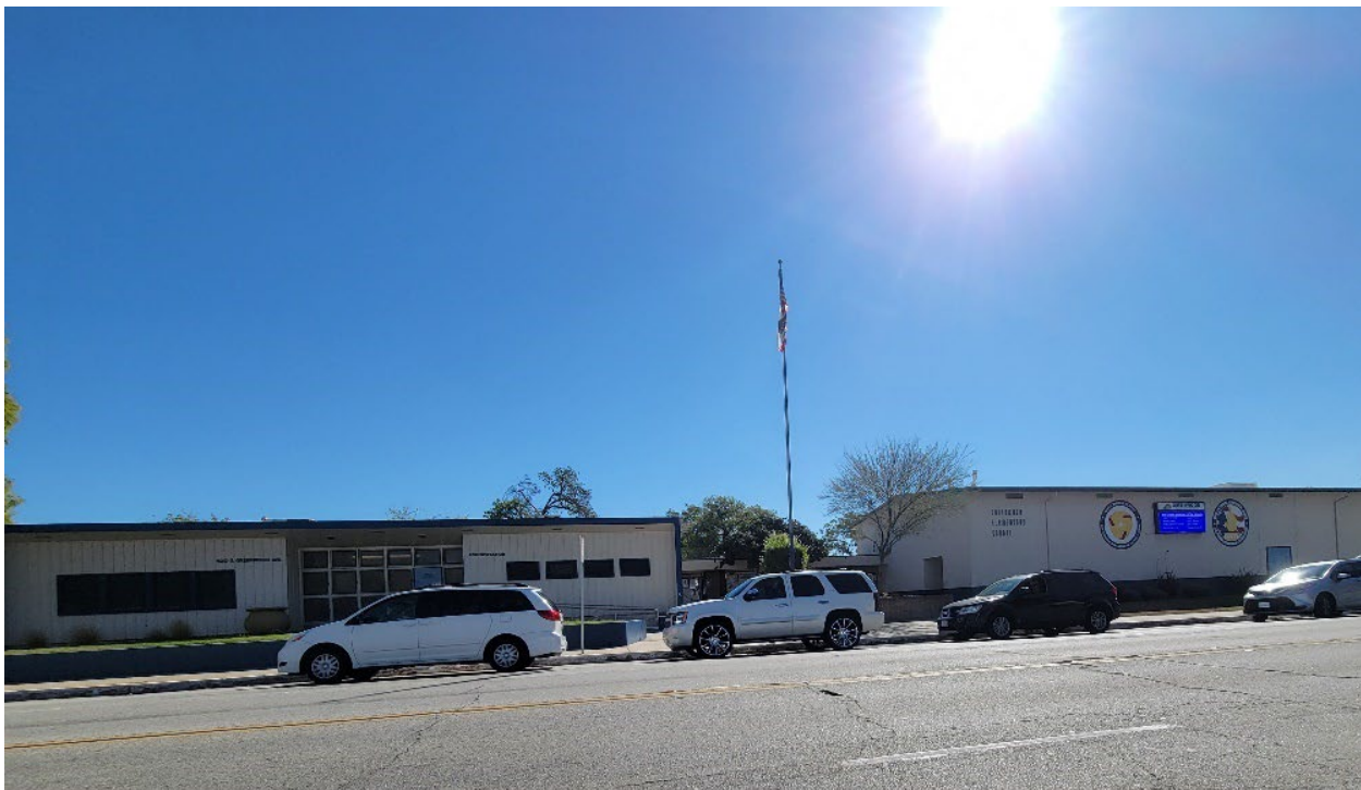
Figure 3.4.7. Greenwood Elementary School Constructed 1947 (900 South Greenwood Avenue) (View east)
