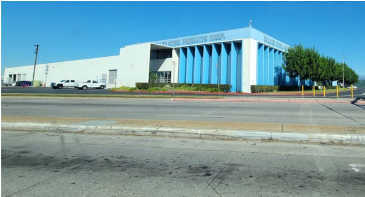
Figure 3.4.5. Pacific Metals Company Building Constructed 1955 (2187 Garfield Avenue) (View northwest)
