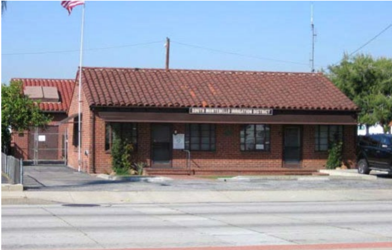
Figure 3.4.8. South Montebello Irrigation District Building Constructed 1940 (864 Washington Boulevard) (View north)
