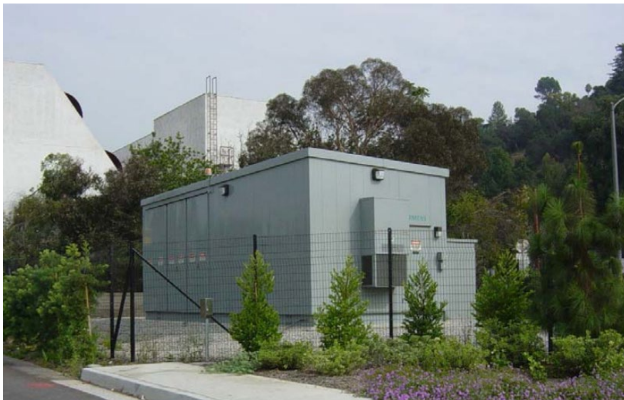
Figure 2.23. Typical Light-Rail TPSS
