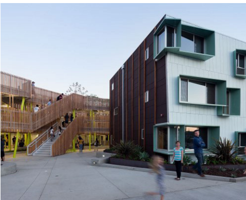
Figure 35 Broadway Housing in Santa Monica makes use of setbacks to create open space and circulation.
