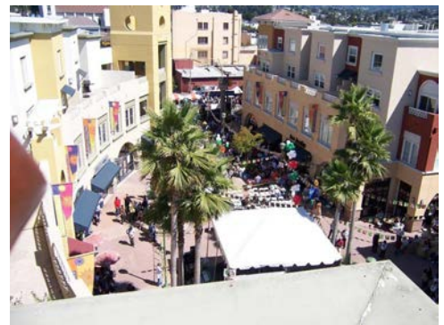
Figure 34 Fruitvale Village is a mixed-use transit-oriented development adjacent to the BART Station in Oakland, CA. The building is oriented to and faces a pedestrian plaza which hosts farmer's markets and events.
