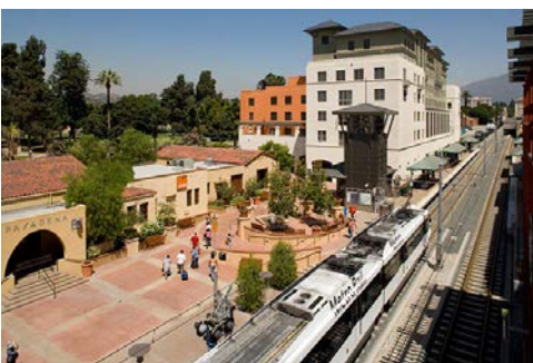
Figure 36 Transit plaza of Del Mar Station Transit Village, located at the southern edge of downtown Pasadena, along the Gold Line.
