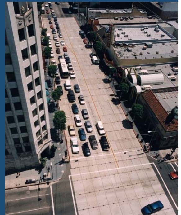
Concrete decking along Hollywood Blvd. during Red Line Construction
