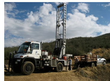
Rotary Wash Drill Rig
