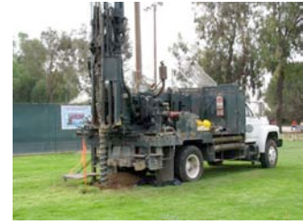
Continuous Core Drill Rig
