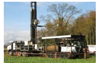
Sonic Core Drill Rig
