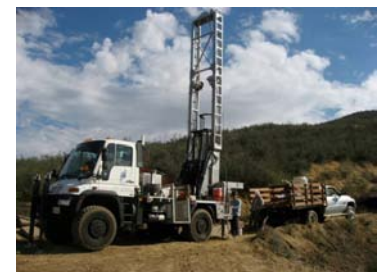
Rotary Wash Drill Rig
