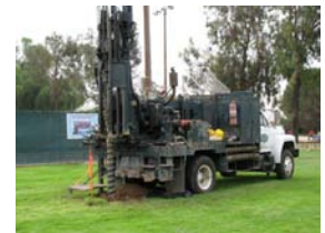
Continuous Core Drill Rig
